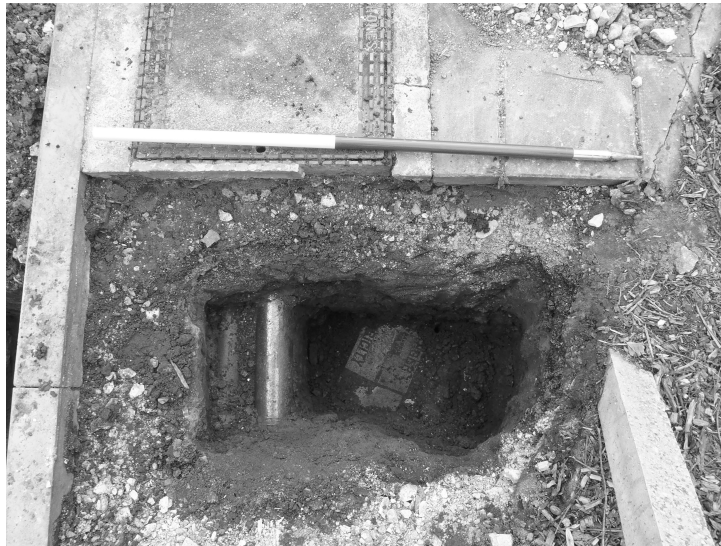
Plate 3 - Trench 2b, looking south, 1m scale
