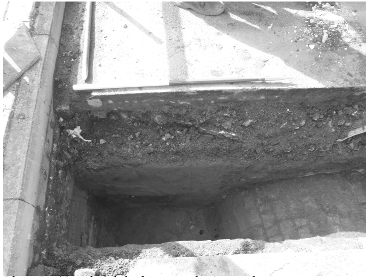
Plate 5 - Trench 2d, looking south, 1m scale
