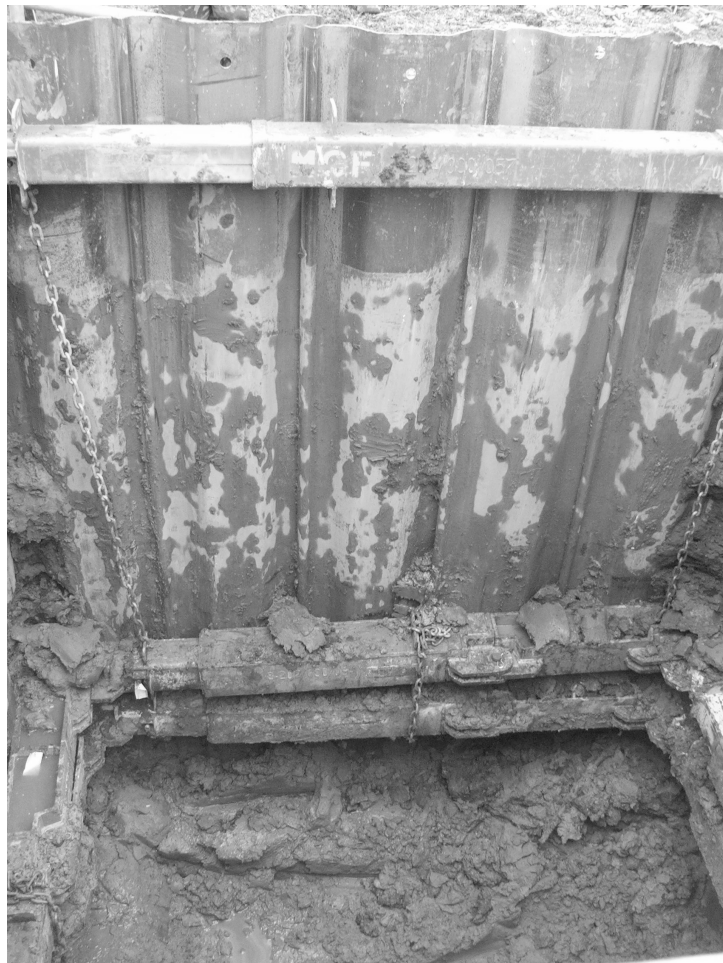
Plate 1 - Depth of excavation, looking west
