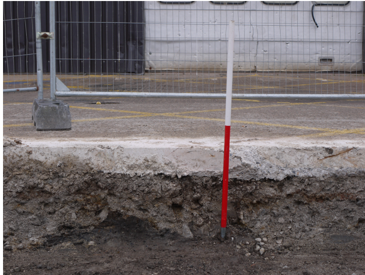
Plate 2 - Car Park make up, looking south. 1m scale
