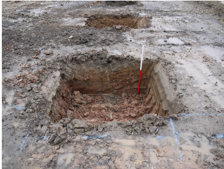
Plate 3 - Foundation pad excavation, looking west. 1m scale
