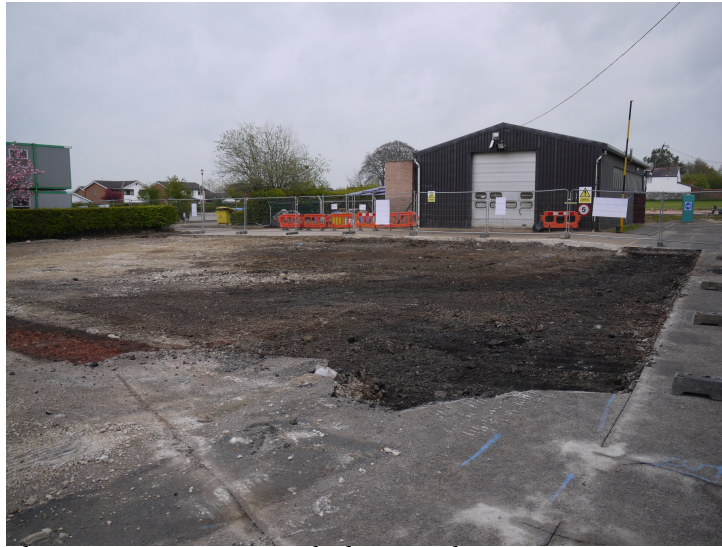
Plate 1 - Excavation area, looking southeast
