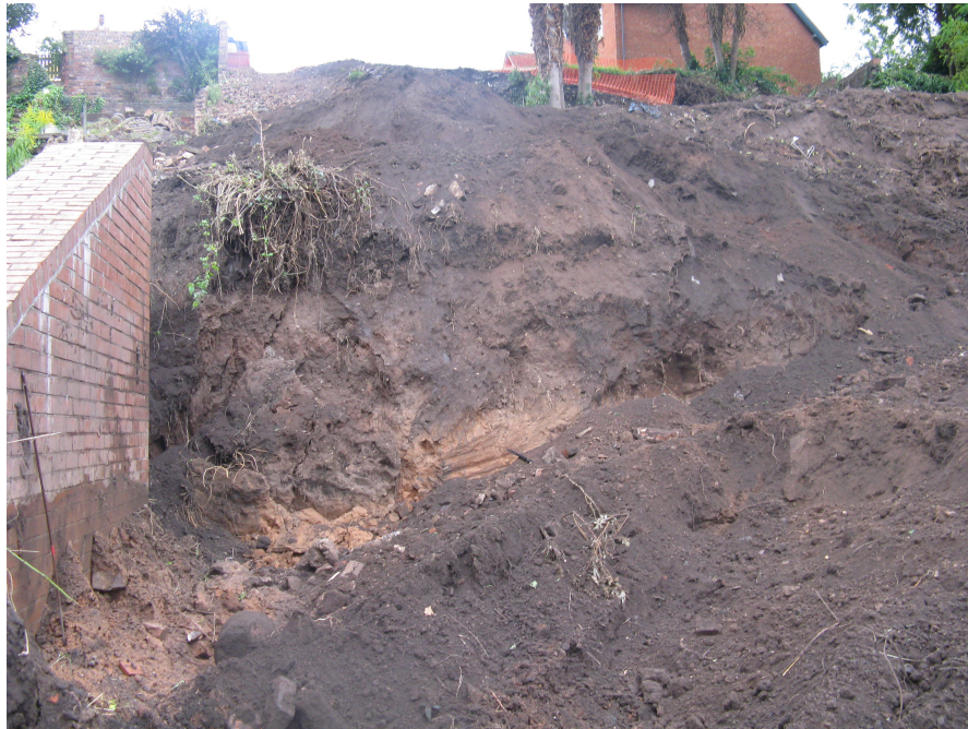
Plate 2 - Section 2, looking west.
