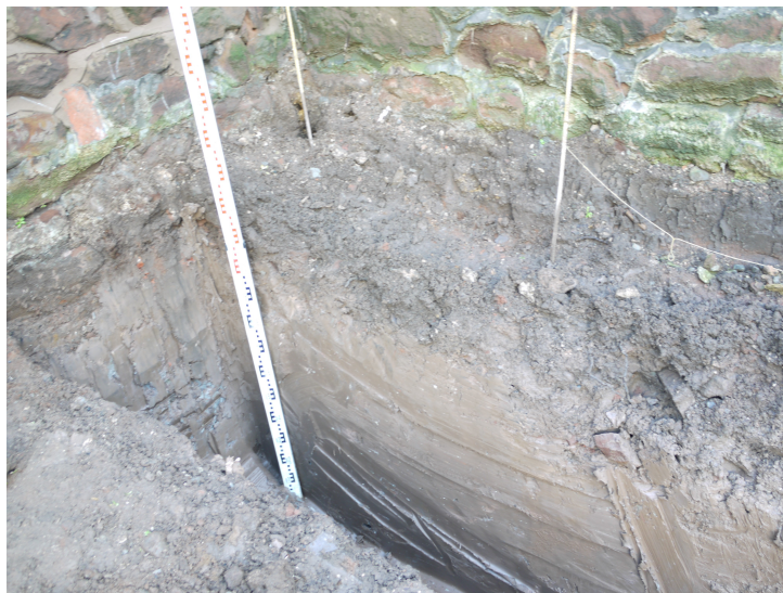
Plate 1 - Southwest facing section of footing excavation
