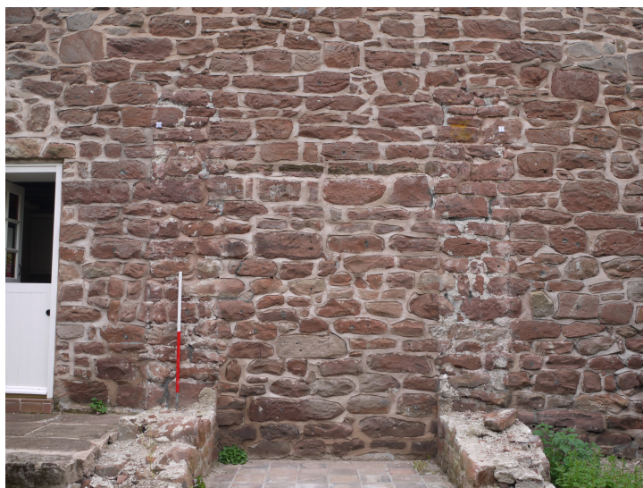
Plate 3 - Ghosting for buttresses on southwest elevation, 1m scale
