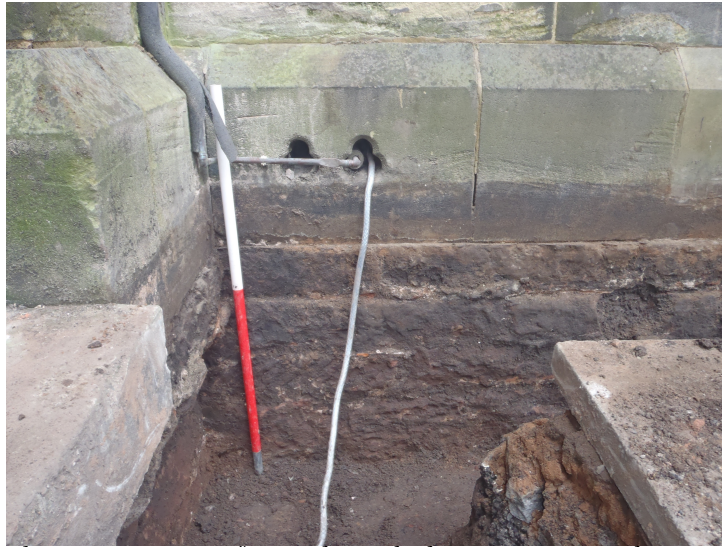
Plate 4 - Footings of St Andrews, looking west, 1m scale
