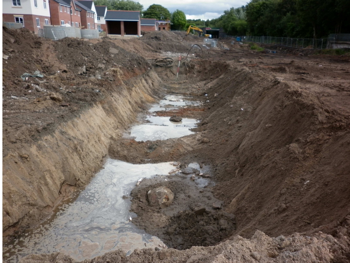
Plate 5: Trench 7, looking north, 2m scale
