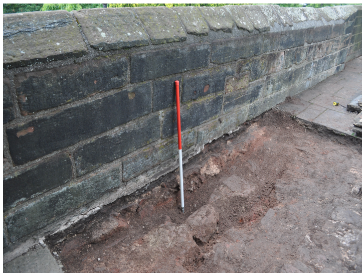
Plate 10: Section of Works looking South-East, 1m Scale
