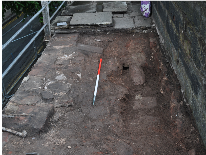
Plate 9: Wall Excavations looking North, 1m scale
