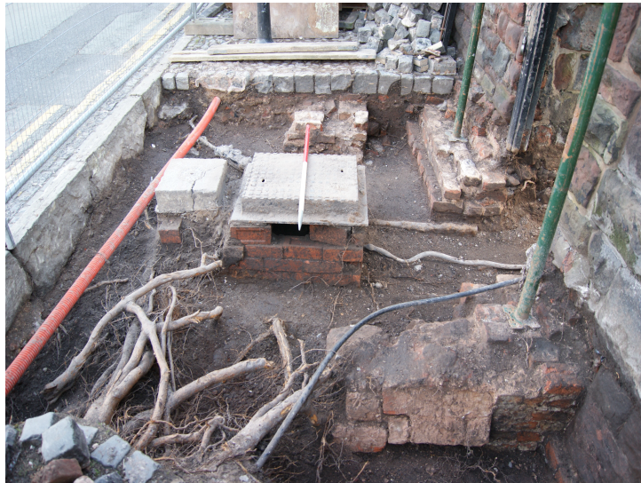
Plate 7: Western Side looking North, 1m Scale
