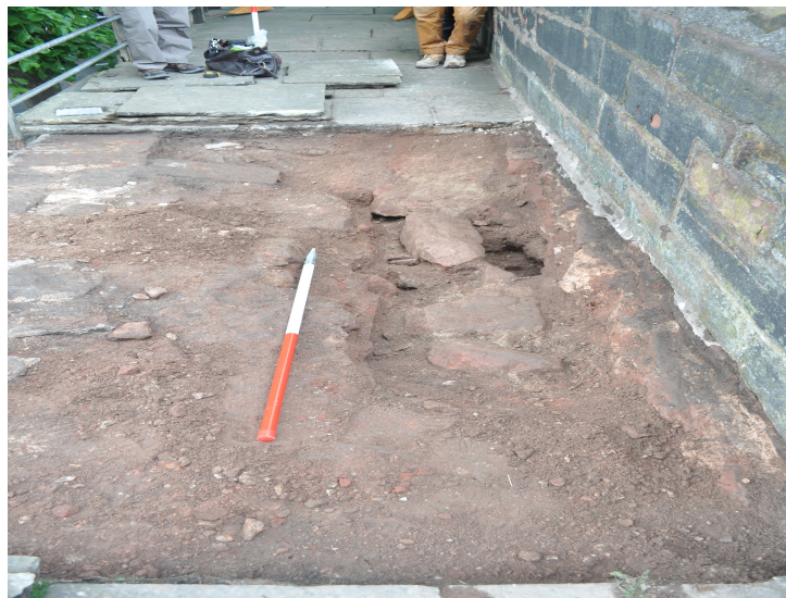
Plate 11: Full extent of works looking North, 1m scale
