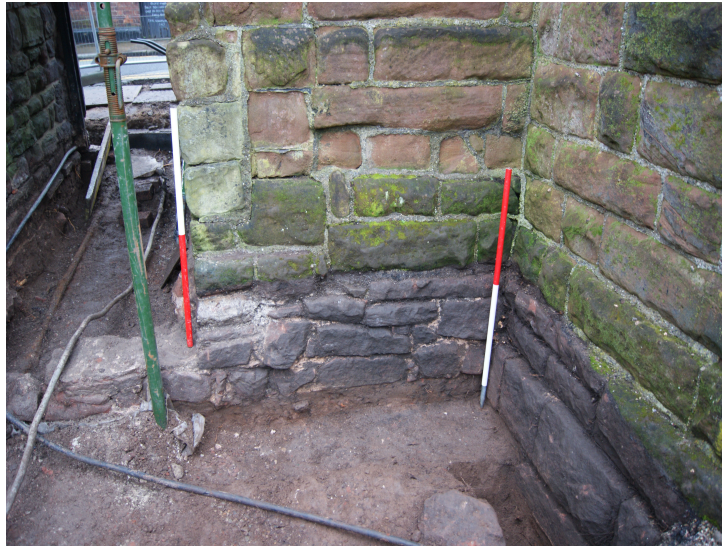
Plate 2: Entranceway looking West, 2x1m Scale
