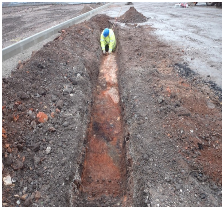
Plate 1 - View of trench 1 Looking north-east.
