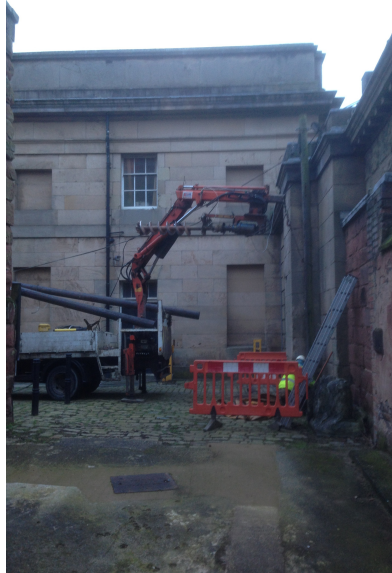
Plate 1 - Photograph showing arm and chain set-up for removal of pole
