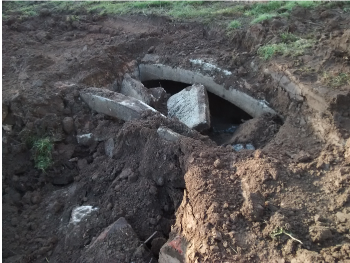
Plate 1 - Concrete culvert (07) with rubble infill
