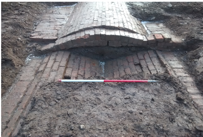
Plate 2 - Culvert looking southeast showing collapse (03), arch (05) and culvert (06). 1m scale.
