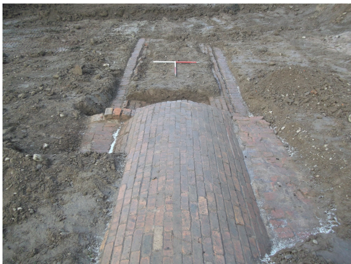
Plate 3 - Culvert looking southeast. Natural geology to right of structure. 2 x 1m scale
