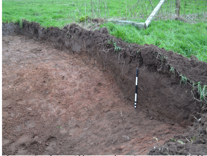
Plate 4: Trench one: Oblique northeast facing section of field boundary, Facing South, 0.5m scale
