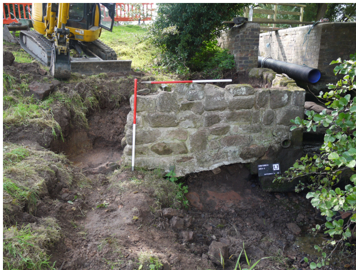
Plate 3: North facing elevation of sluice, 2 x 1m scales.
