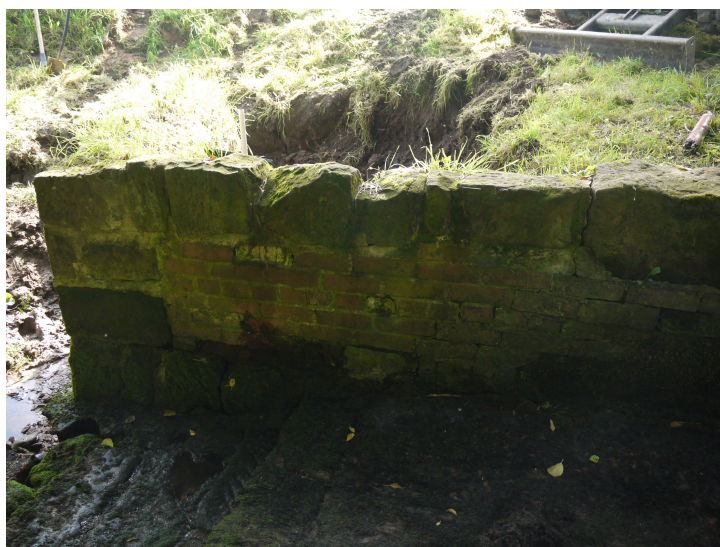
Plate 4: Inner face of sluice wall, looking east.
