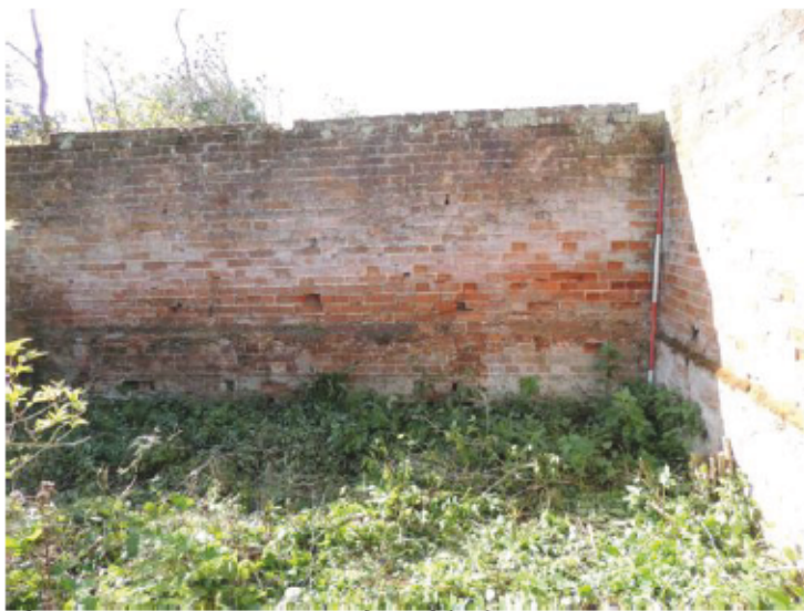
Plate 14 - Structure 3 South End looking west
