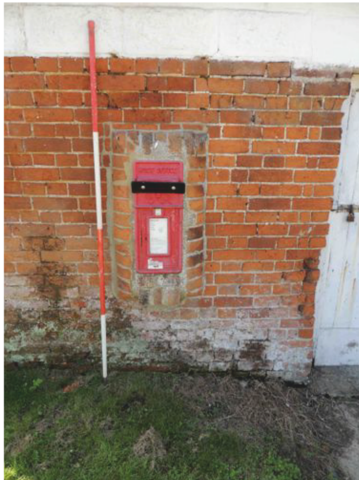
Plate 28 - Structure 6 Letterbox Detail looking west
