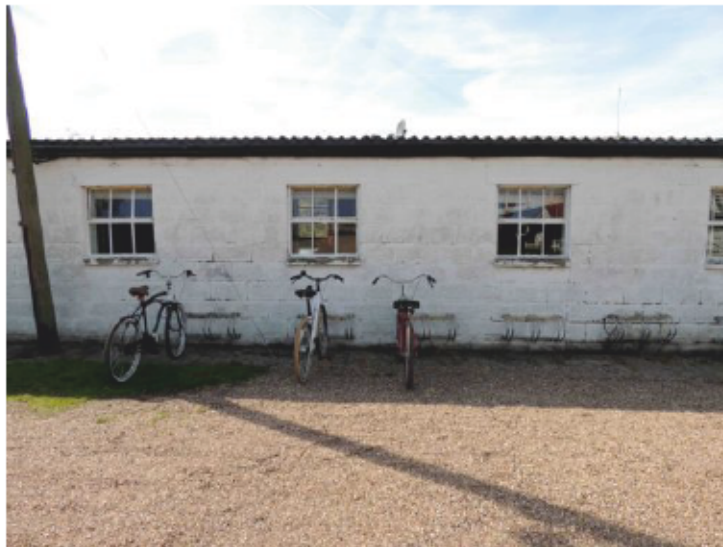
Plate 26 - Structure 6 East Elevation Middle looking west
