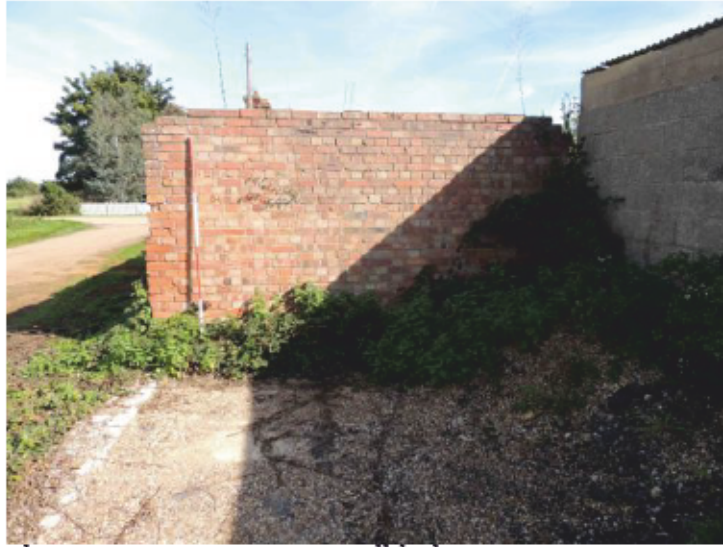
Plate 19 - Structure 5 West Wall looking east
