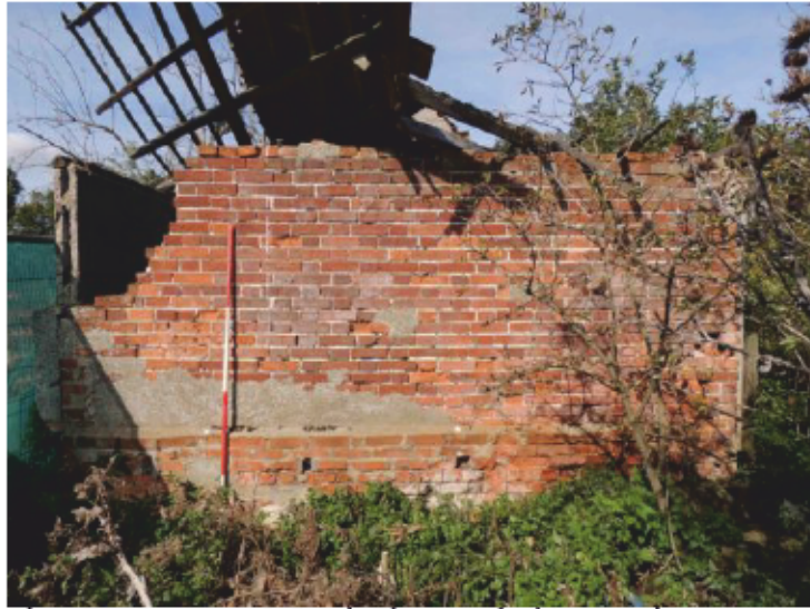
Plate 7 - Structure 2 South Elevation looking north
