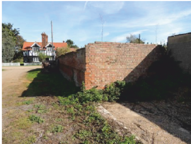
Plate 18 - Structure 5 looking east
