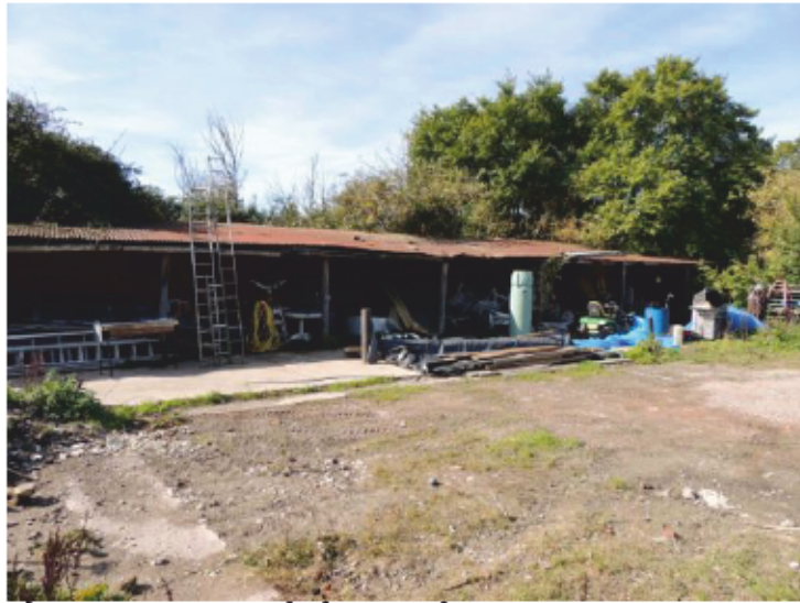
Plate 1 - Structure 1 looking northwest
