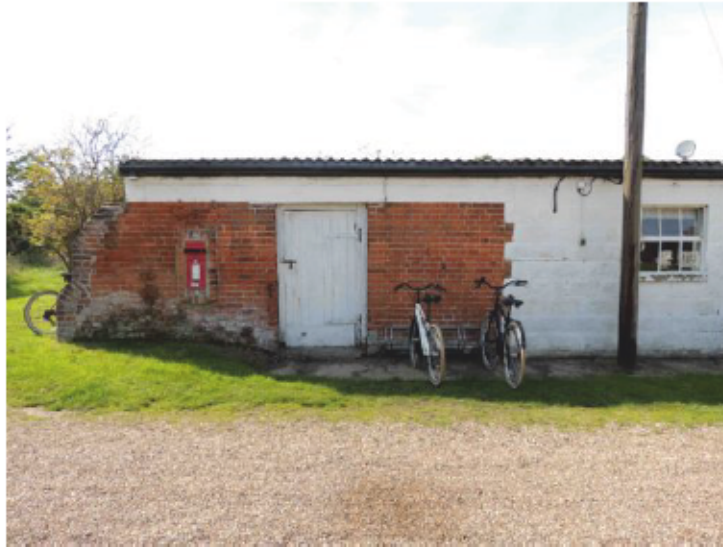
Plate 27 - Structure 6 East Elevation South End looking west
