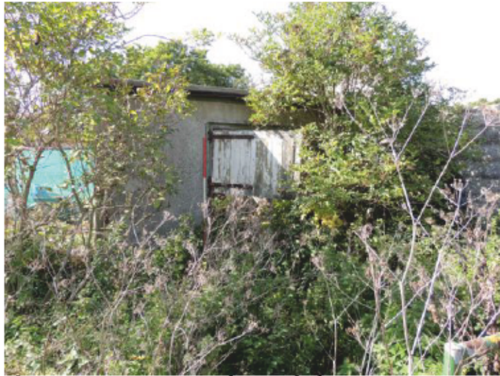
Plate 6 - Structure 2 East Elevation looking west
