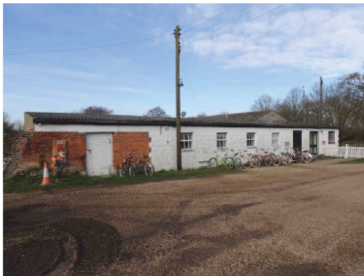
Plate 22 - Structure 6 looking north west
