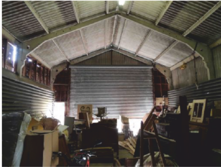
Plate 43 - Structure 7 Internal looking west
