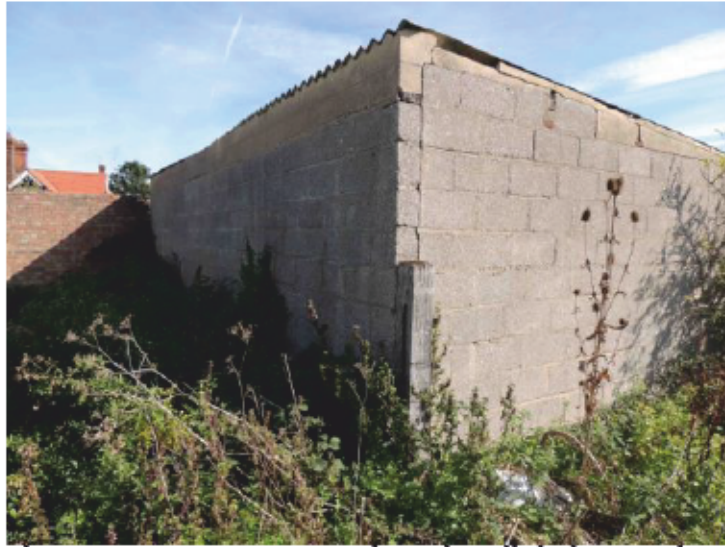
Plate 17 - Structure 4 West and North Walls looking south east
