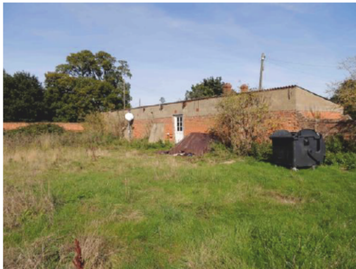
Plate 30 - Structure 6 West Elevation looking north east
