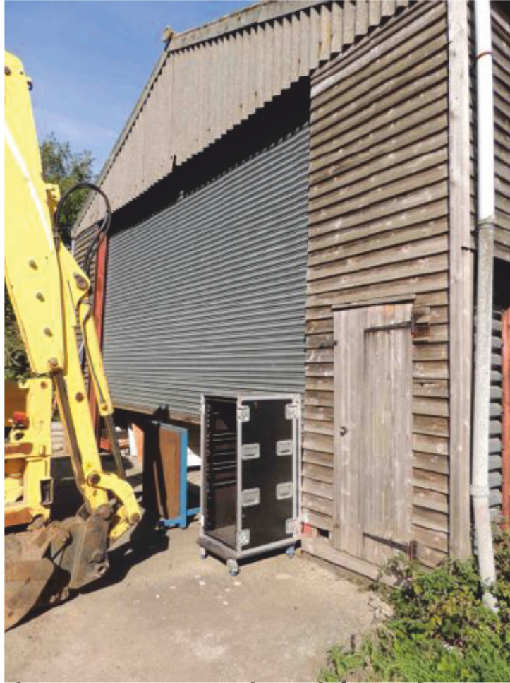
Plate 41 - Structure 7 West Elevation looking north
