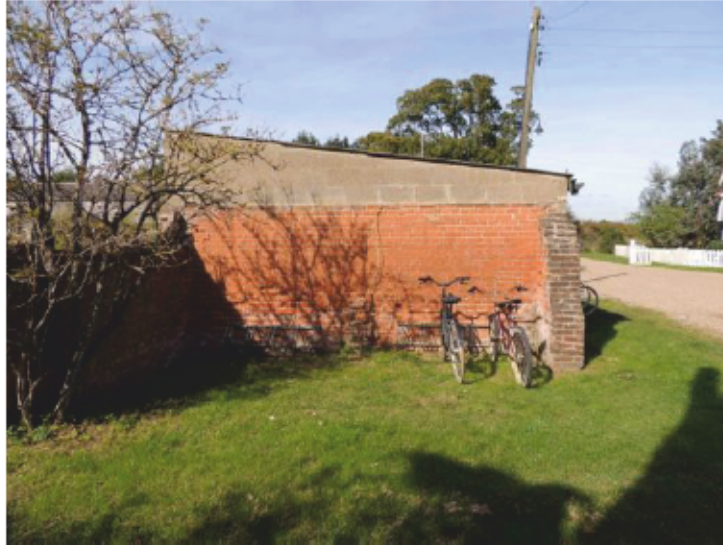
Plate 29 - Structure 6 South Elevation looking north
