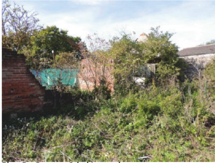
Plate 5 - Structure 2 looking north west
