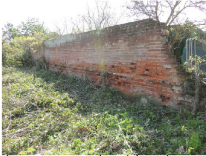
Plate 11 - Structure 3 East Elevation looking south west
