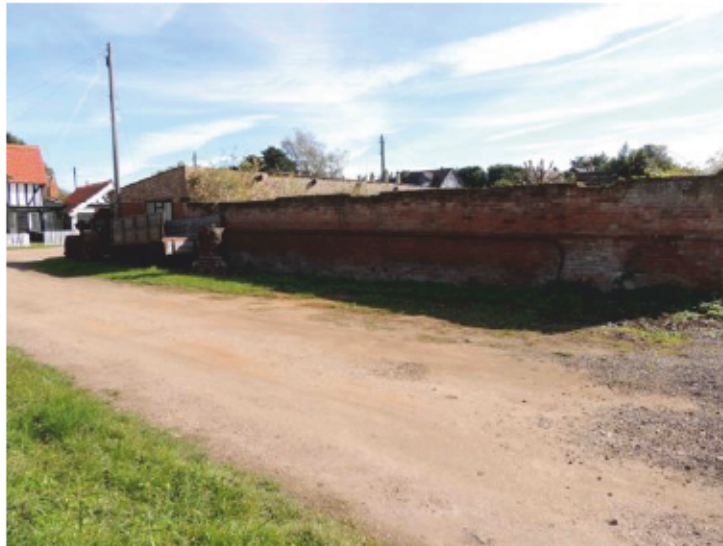
Plate 20 - Structure 5 North Wall looking south east
