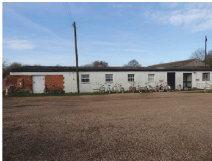
Plate 24 - Structure 6 East Elevation looking west
