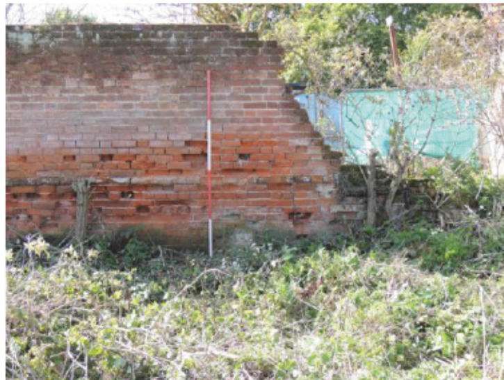
Plate 12 - Structure 3 North End looking west
