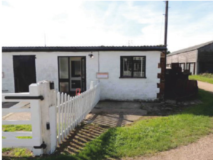
Plate 25 - Structure 6 East Elevation North End looking west
