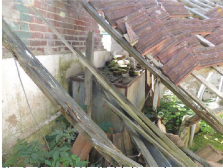
Plate 9 - Structure 2 Metal Tank looking south west
