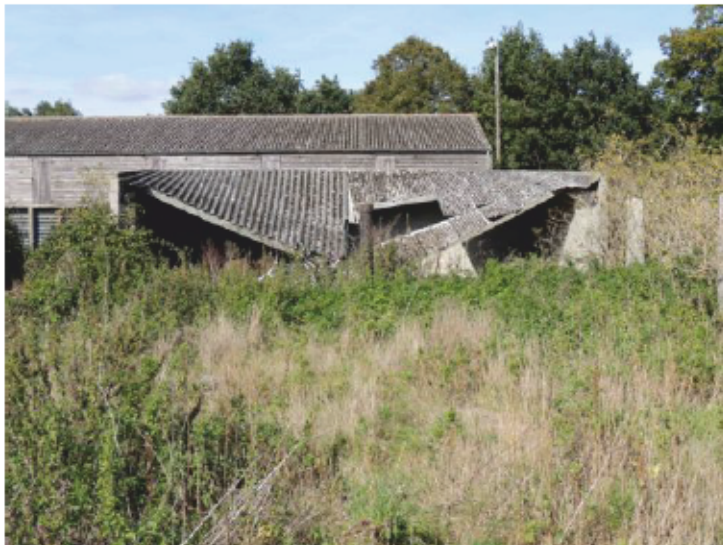
Plate 16 - Structure 4 looking north
