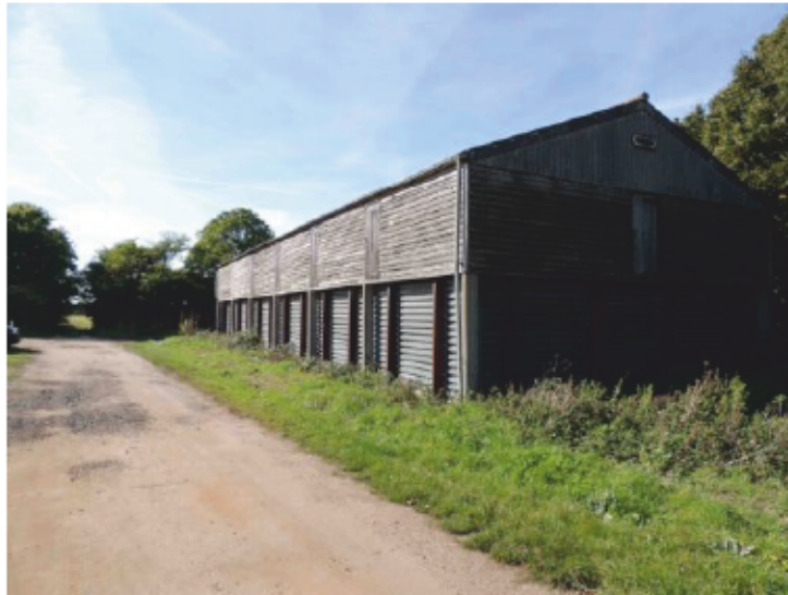
Plate 40 - Structure 7 looking west
