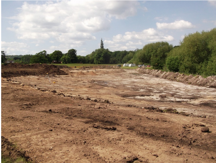
Plate 1 - Stripped area looking NW
