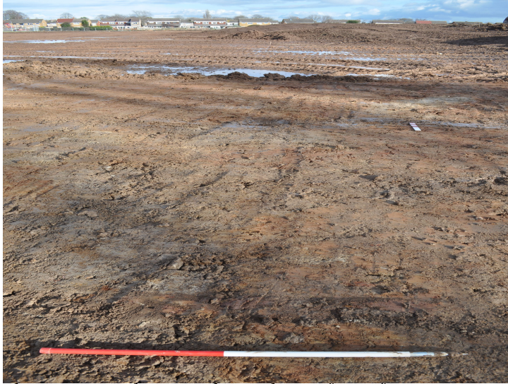
Plate 4: Stripped area to the northeast of site, facing east. 1m scale.
