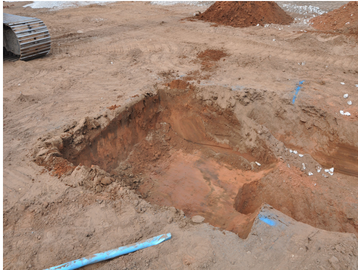
Plate 2: Exposed area of [12], looking south.
