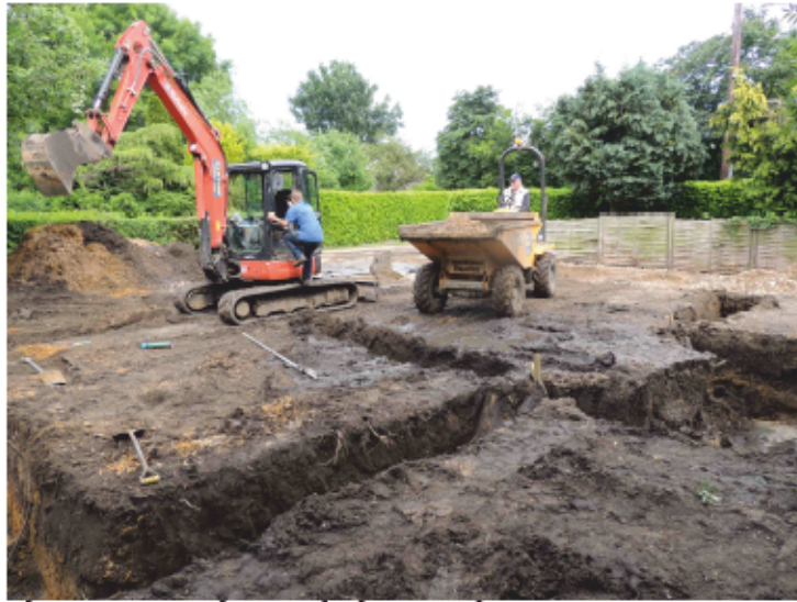
Plate 1 - General View, looking northeast
