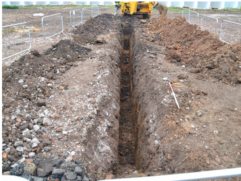
Plate 2 - Shot of excavation for groundworks, looking north
