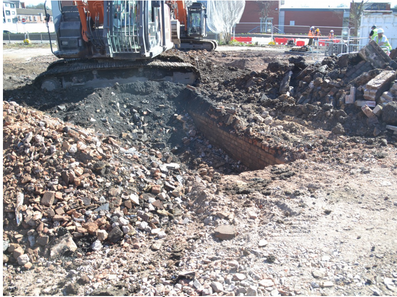
Plate 1 - Continuing groundworks on site
