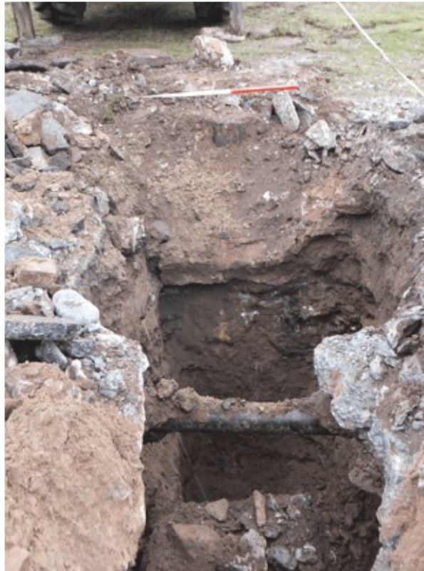
Plate 2 - The vertical south west facing section of the Sea wall in TP104A
