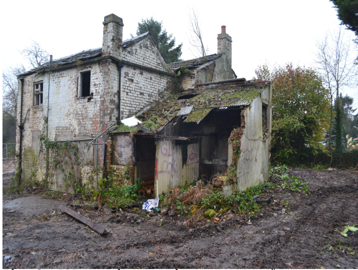
Plate 3 - Western elevation, showing twin roof structure
