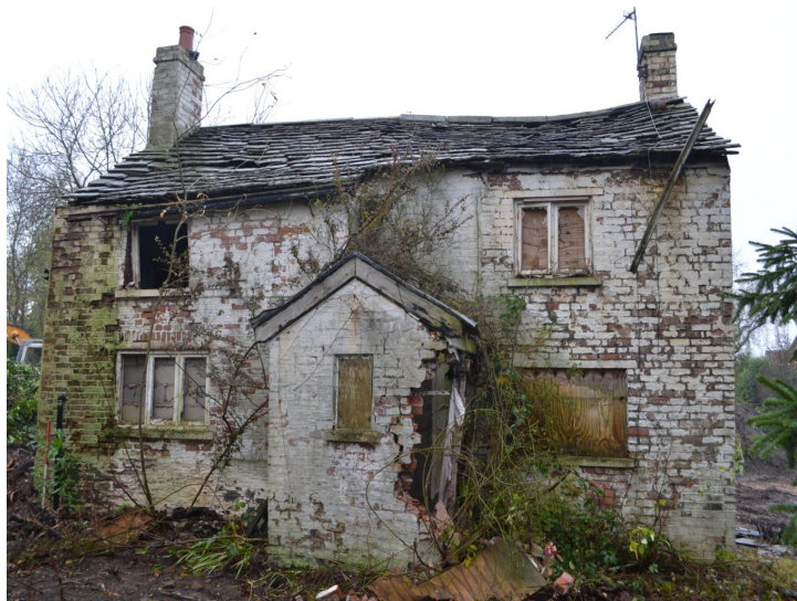
Plate 1- South facing elevation
