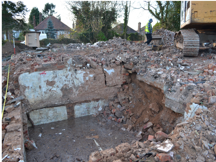
Plate 10 - Cellar east wall
