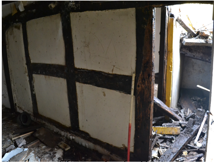
Plate 7 - Ground floor exposed cruck and box frame
