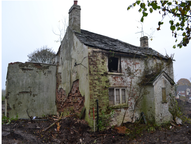
Plate 2 - Southern elevation, from the west
