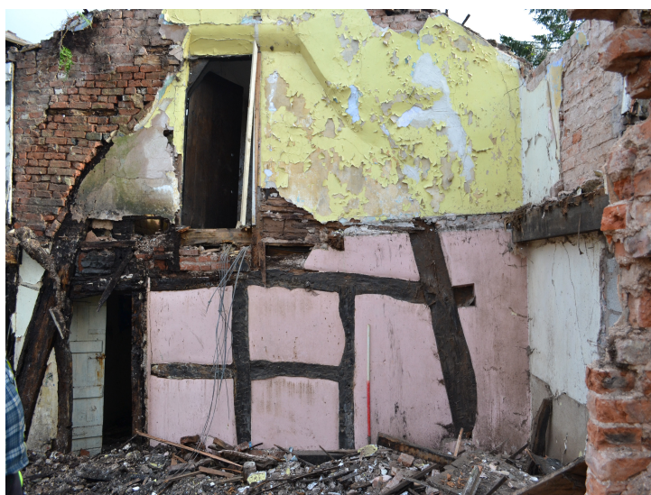
Plate 6 - Cruck frame on central wall of southern block
