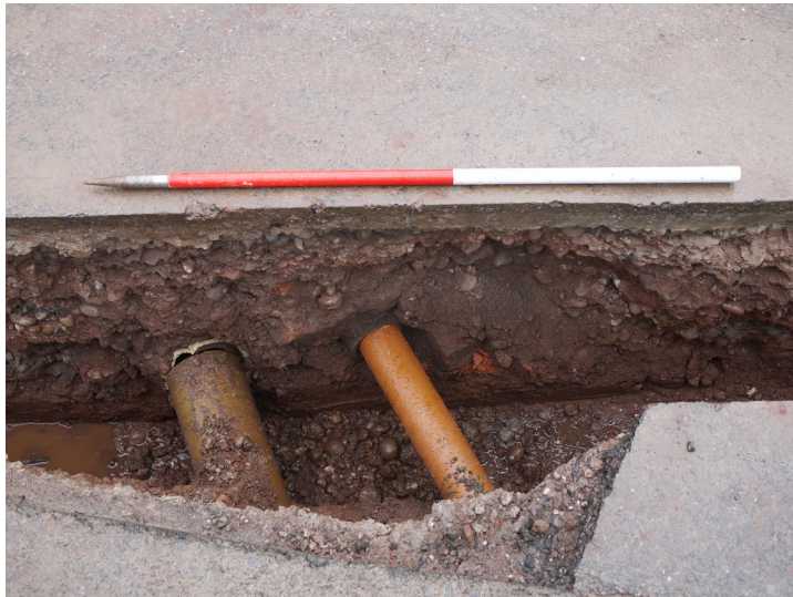
Plate 9 - West facing section with exposed drainage pipes, with 1m scale
