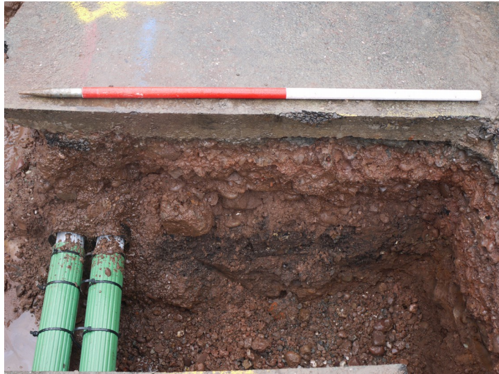
Plate 10 - South facing section with exposed pipes, with 1m scale
