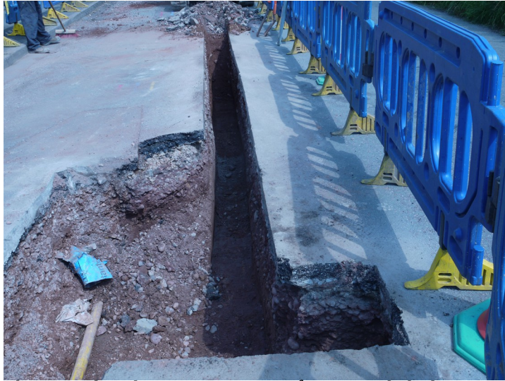
Plate 5 - Shot showing excavation of pipe trench, looking north
