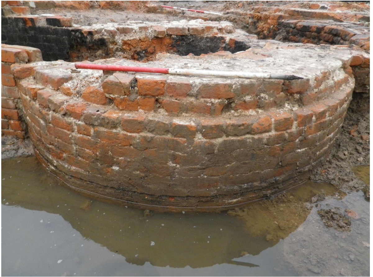
Plate 12 - Trench 1. Looking north-west showing the elevation of Chimney wall (58), 1 x 1m scale.
