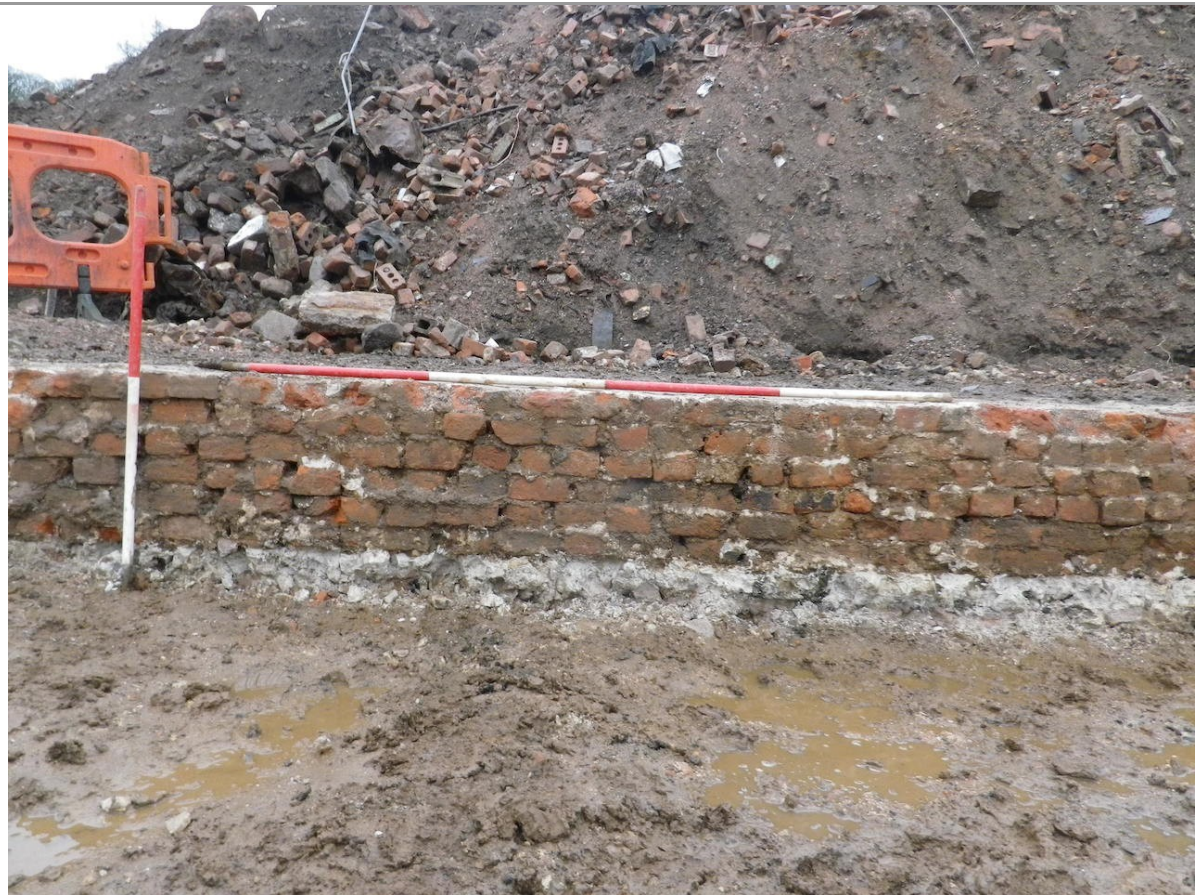
Plate 5 - Trench 4. Looking west, showing the mortar and brick wall elevation of Carding Room wall foundation (14), 1 x 1m and 1 x 2m scale.
