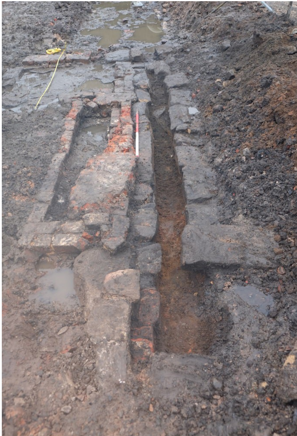
Plate 21 - Trench 2. Looking south-west showing the eastern end of stone culvert (103), 1 x 1m scale.
