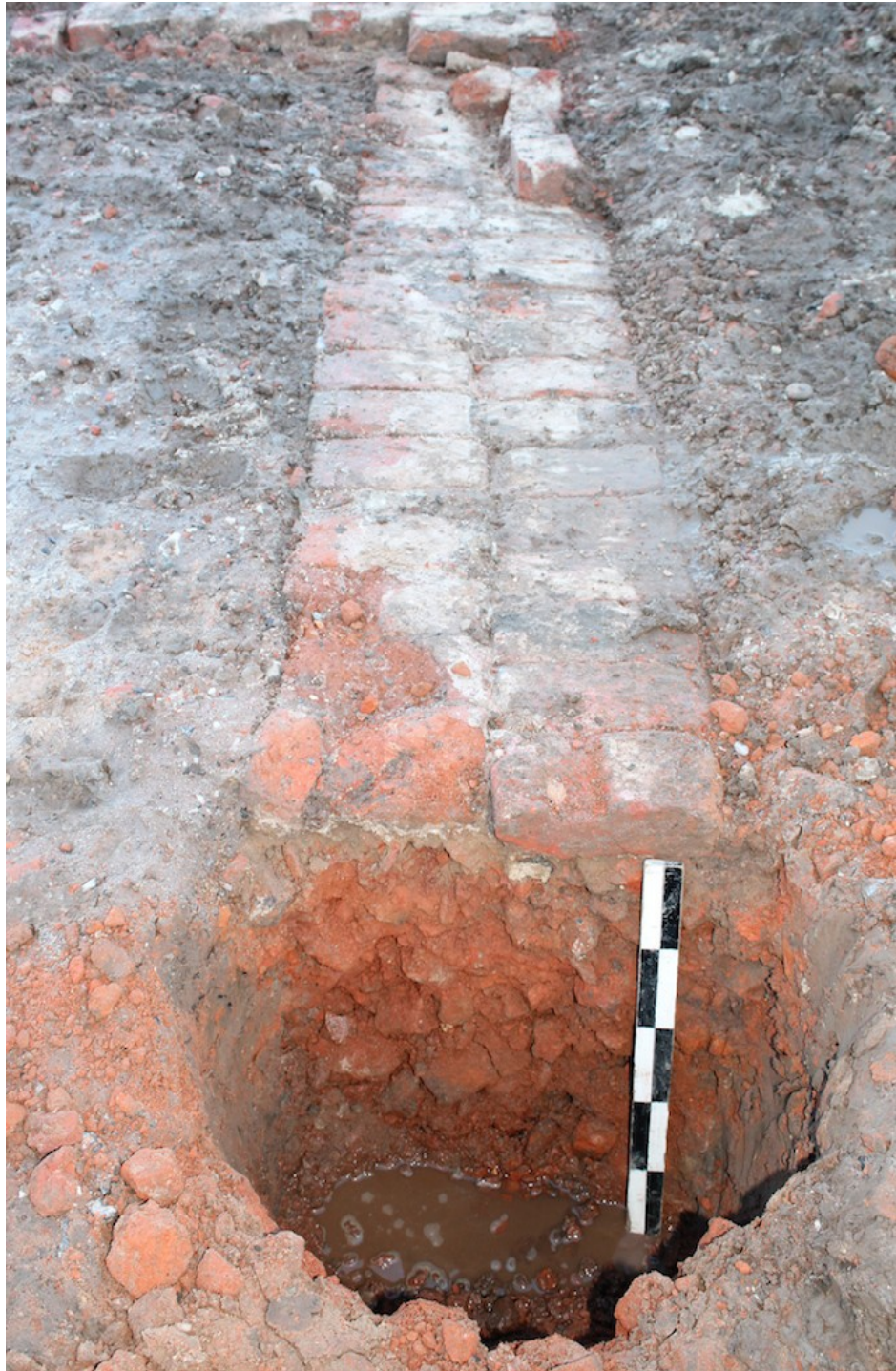
Plate 22 - Trench 2. Looking north-east showing the brick rubble foundation trench to wall (86), 1 x 0.5m scale.
