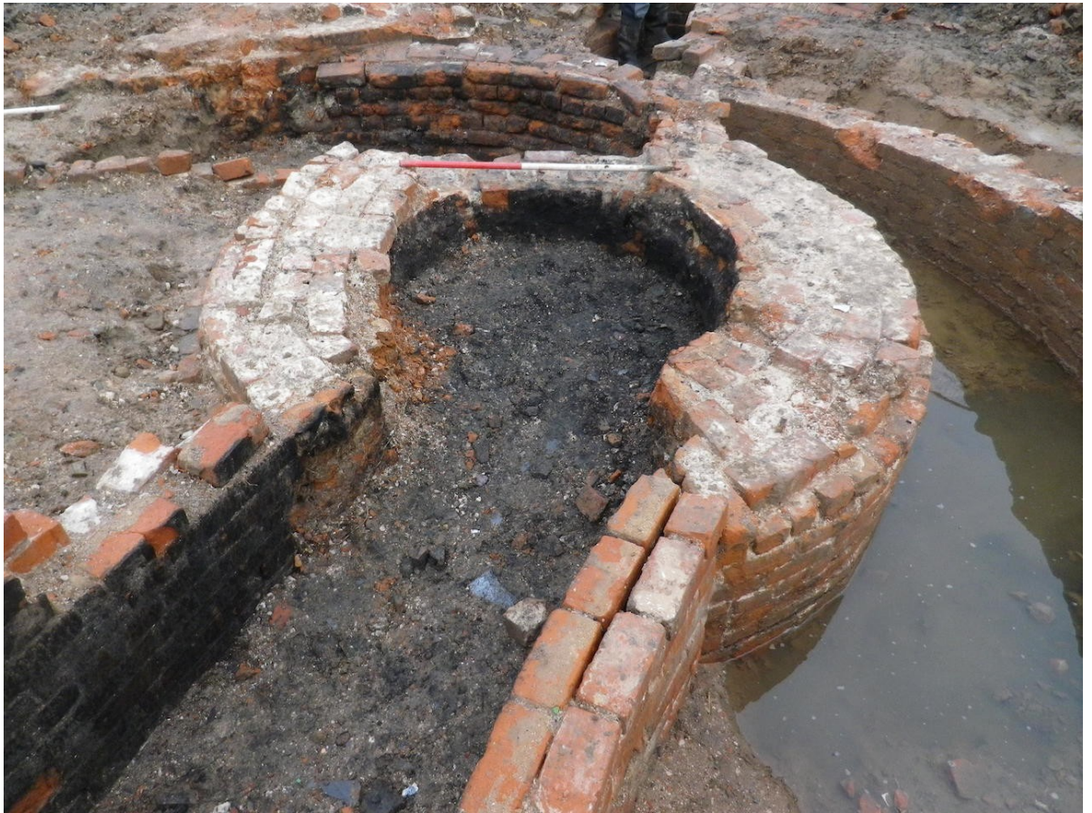
Plate 18 - Trench 1. Looking north-east showing Phase 5 flue walls (49)/(51) and blocking wall to Phase 3 flue, 1 x 1m scale.
