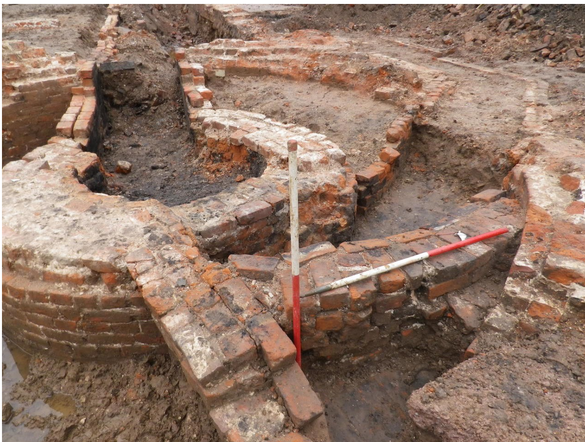
Plate 14 - Trench 1. Looking north-west showing the elevation of flue blocking wall (59), 2 x 1m scale.
