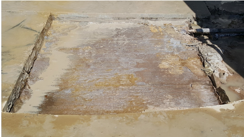
Plate 5 - Shot of concrete base below flagstones
