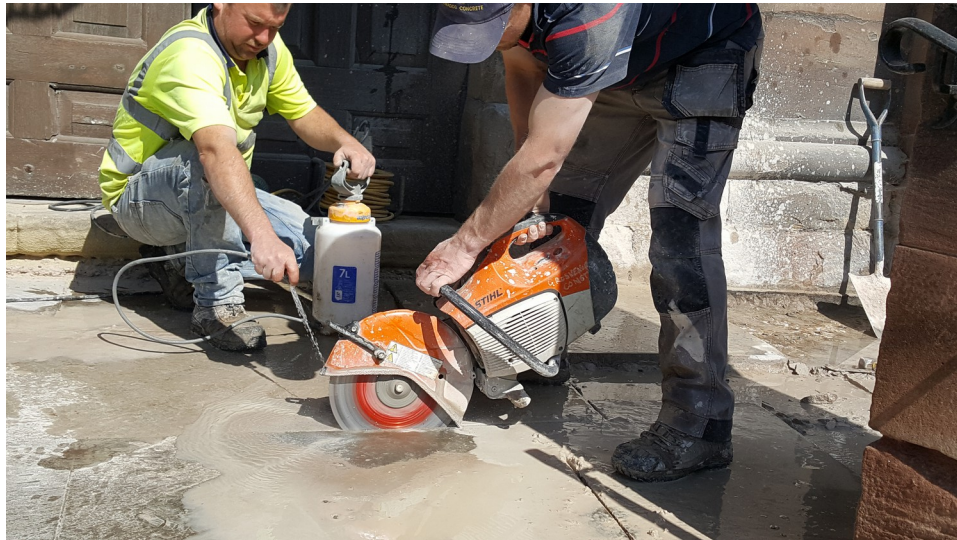
Plate 3 - Working shot of Stihl saw being used to cut the mortar
