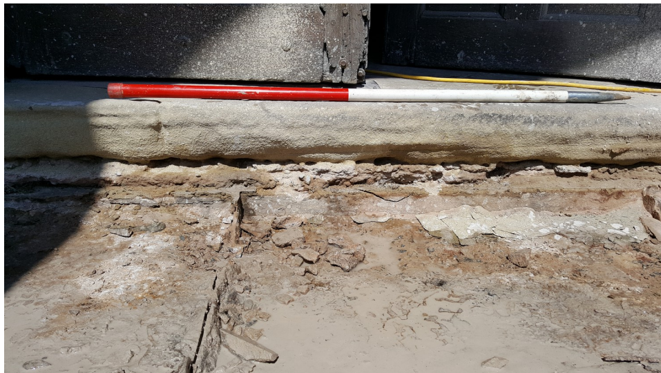
Plate 4 - East facing section of flagstones below porch columns, with 1m scale
