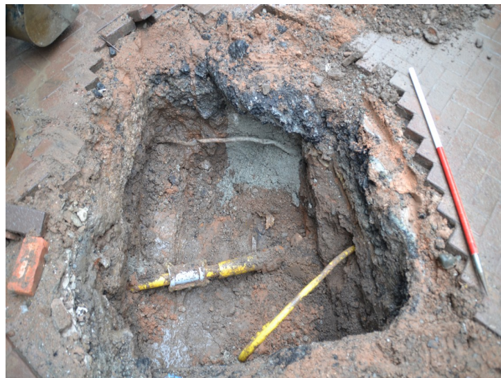
Plate 4 - Overview of Trench 5 with plastic services.
