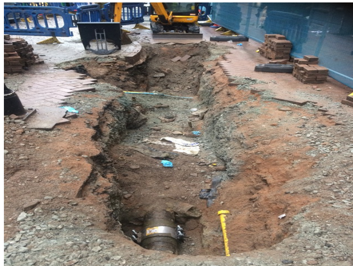
Plate 1 - Working shot of Trench 1 excavation showing gravel fills of services.
