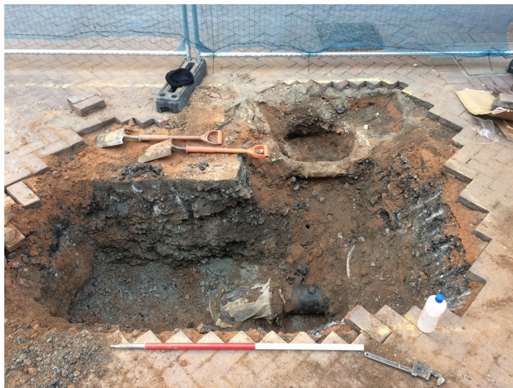
Plate 6 - Trench 7 excavation showing dropping gas main
