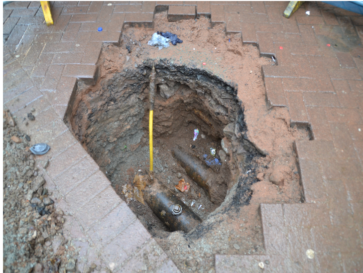
Plate 2 - Trench 2 excavation showing gas mains and adjacent disused mains.
