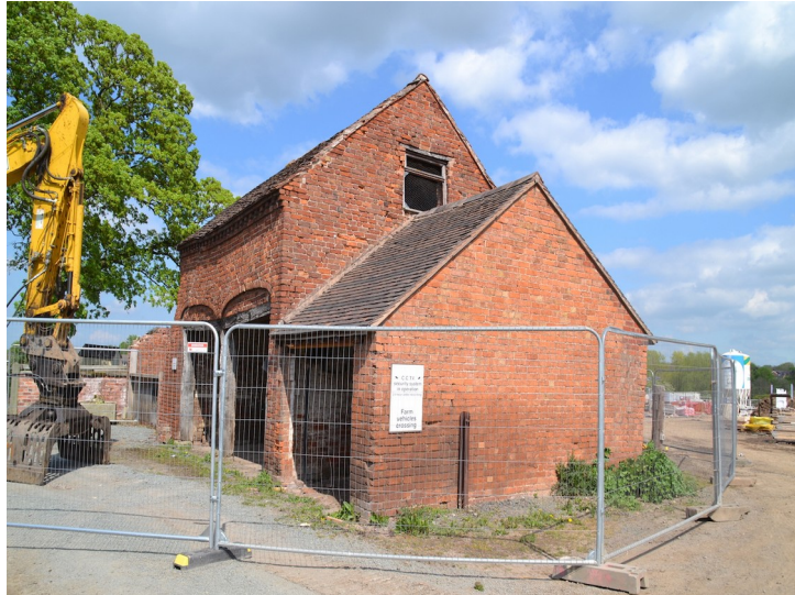
Plate 41- Building G, facing northeast.
