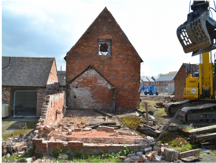
Plate 49- Demolition of building H. Facing east.
