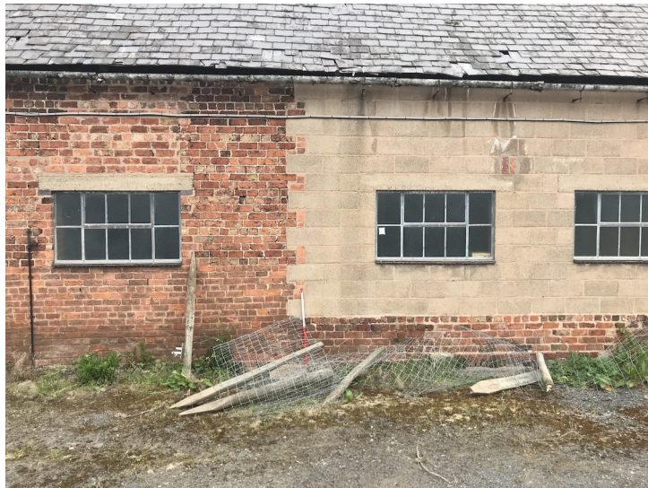
Plate 23- Building E, brick and concrete detail. Facing north, 1m scale.
