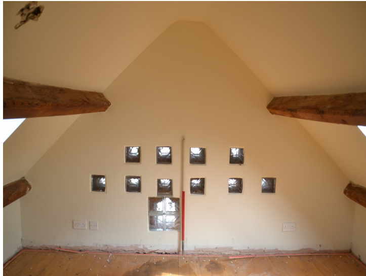
Plate 9- Building B, interior of north elevation, detail of dove holes. Facing north, 1m scale
