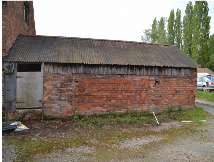
Plate 45- Building H, north facing elevation. Facing south, 1m scale.
