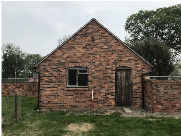
Plate 13- Building C, south facing elevation. Facing north, 1m scale.
