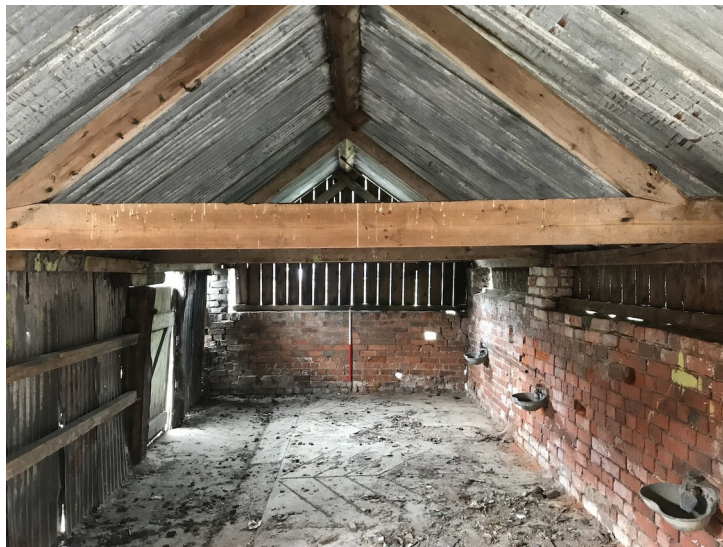
Plate 48- Building H, internal view. Facing west, 1m scale.
