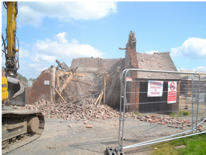
Plate 44- Building G, eastern back wall seen during demolition. Facing east.
