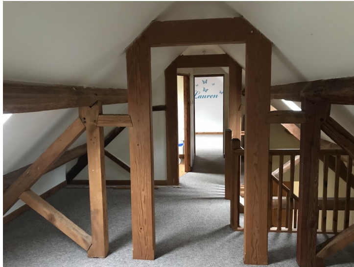
Plate 8- Building B, upper level looking south.
