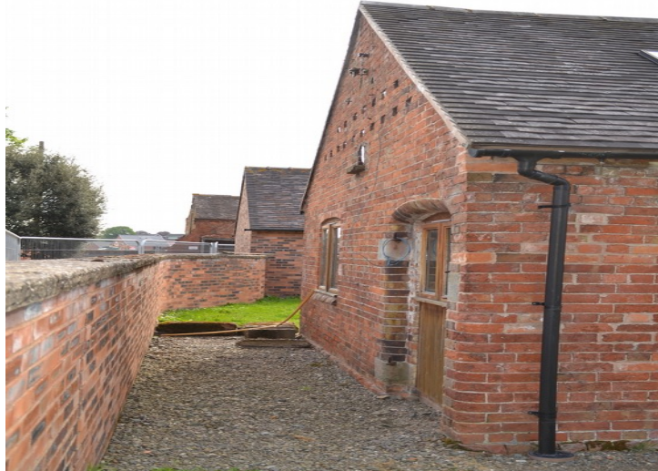
Plate 4- Building B, north elevation. Facing east.
