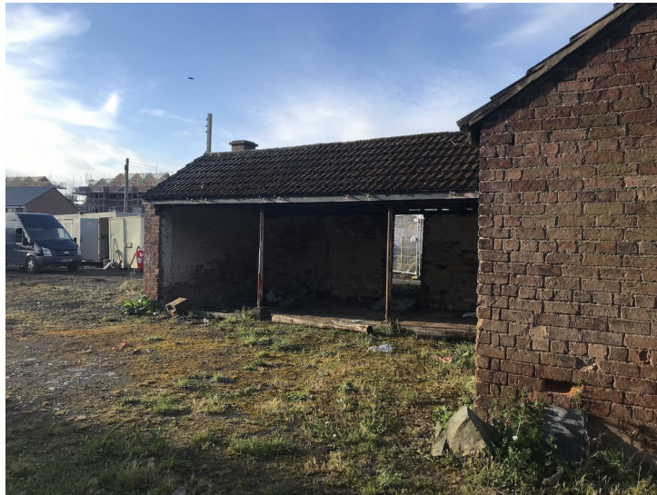
Plate 38- Building F, north open facade. Facing south, 1m scale.
