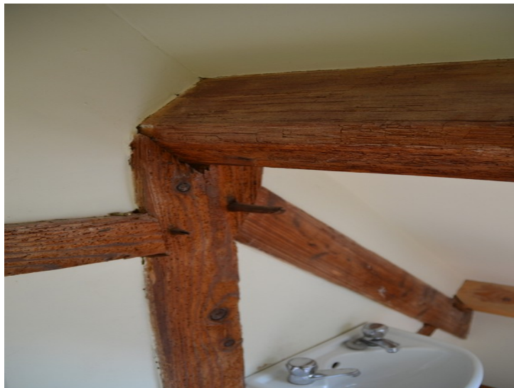
Plate 10- Building B, timber joins in the roof of the upper floor.
