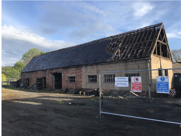
Plate 22- Building E, south and east facing elevations. Facing northwest.
