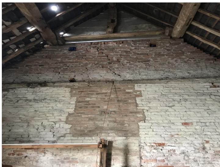
Plate 31- Building E, room 3 brick wall division with blocked up door. Facing west.
