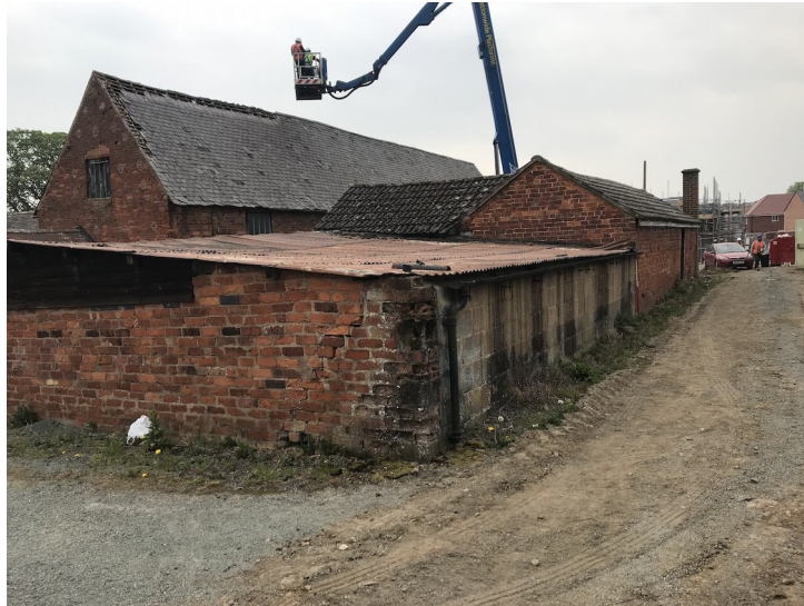
Plate 37- Building F, west and south elevations. Facing northeast.
