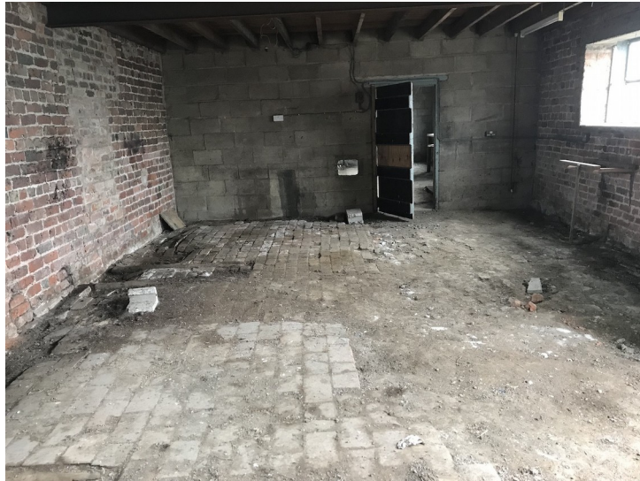
Plate 29- Building E, room 2 facing east.
