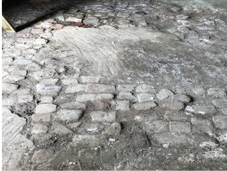
Plate 28- Building E, room 1 concrete and brick floor.
