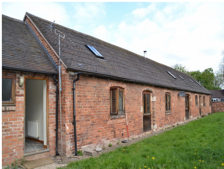
Plate 5- Building B, east elevation. Facing northwest, 1m scale.
