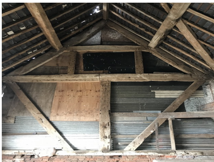
Plate 30- Building E, room 3 exposed wooden beam division, facing east.
