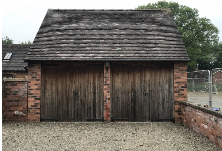
Plate 12- Building C, east facing elevation. Facing west, 1m scale
