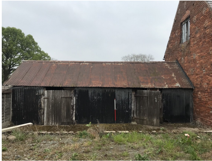
Plate 47- Building H, south elevation. Facing north, 1m scale.
