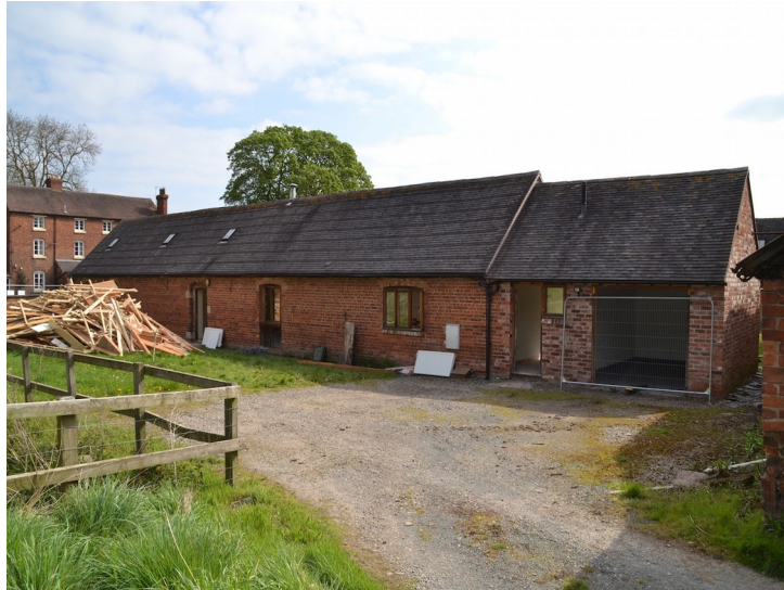
Plate 2- Building B, west elevation. Facing northeast.
