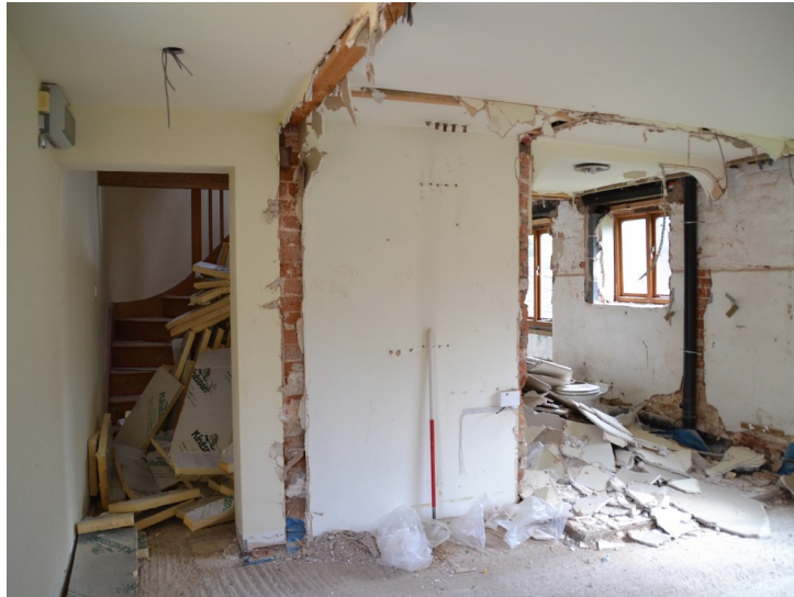
Plate 7- Building B, looking north at staircase. 1m scale
