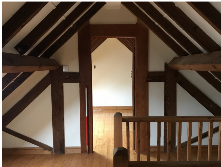
Plate 20- Building D, Upper floor timber beams. Facing north, 1m scale.
