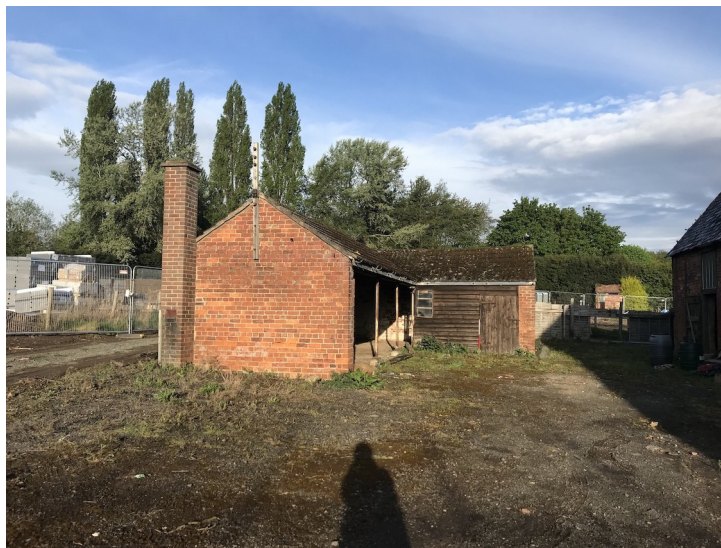
Plate 36- Building F, looking west. 1m scale.
