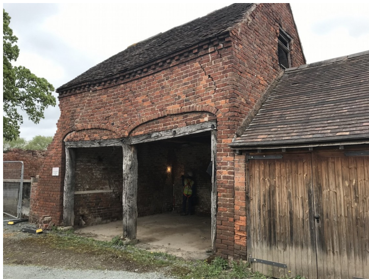
Plate 42- Building G, west facing open frontage. Facing northeast.
