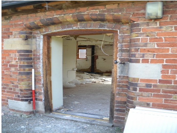
Plate 3- Building B, Door in west elevation. 1m scale
