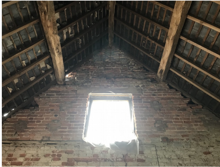
Plate 34- Building E, room 4 internal facade of west external wall. Facing west.
