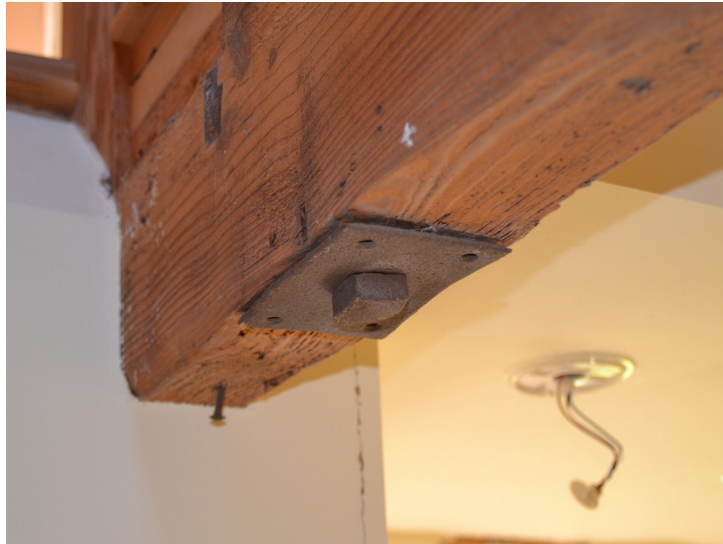
Plate 11- Building B, original iron fixtures, seen on the staircase.
