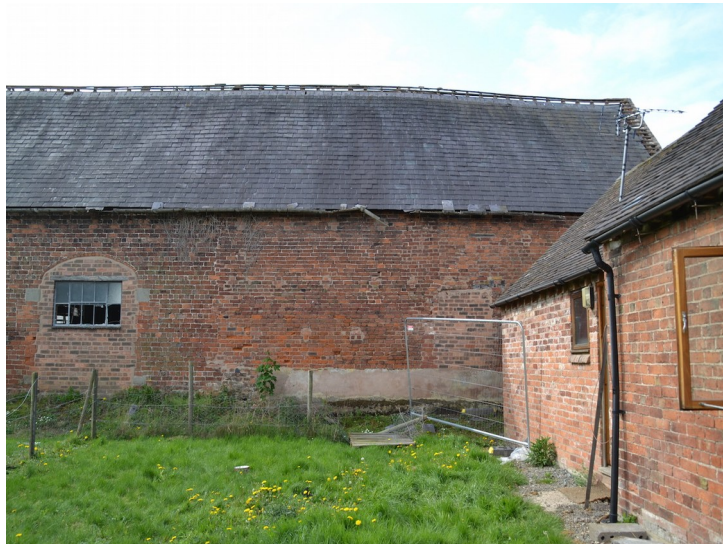
Plate 25- Building E, north facing Elevation. Facing south.
