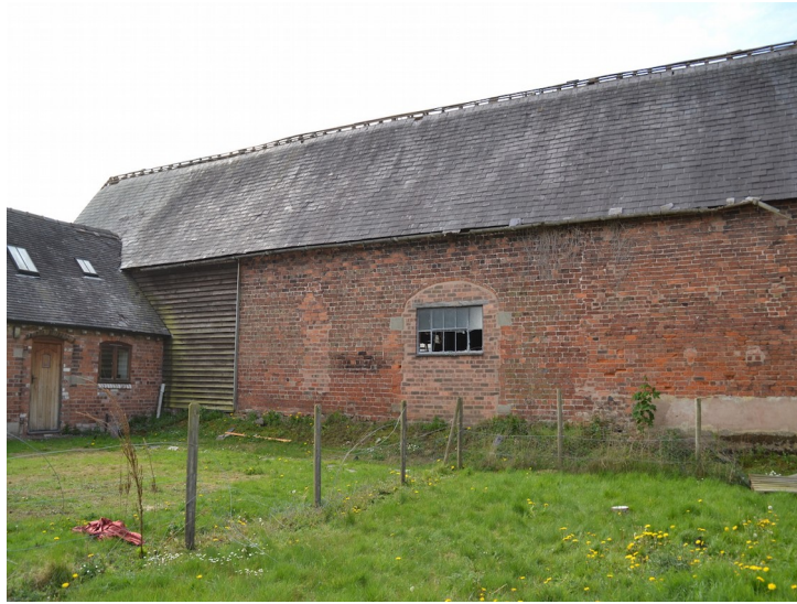
Plate 24- Building E, north facing Elevation. Facing southeast.
