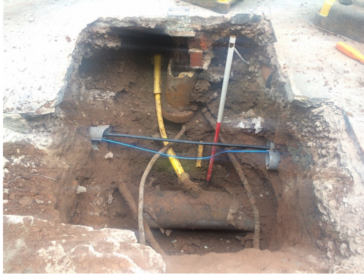
Plate 3- Trench 23 Roshill Bank, facing southwest. 1m scale.
