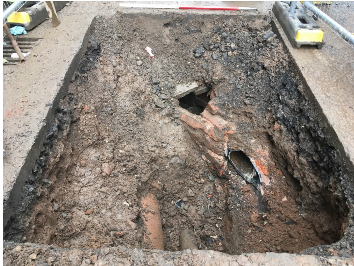
Plate 2- Trench 16, brick culvert (1602).1m scale.
