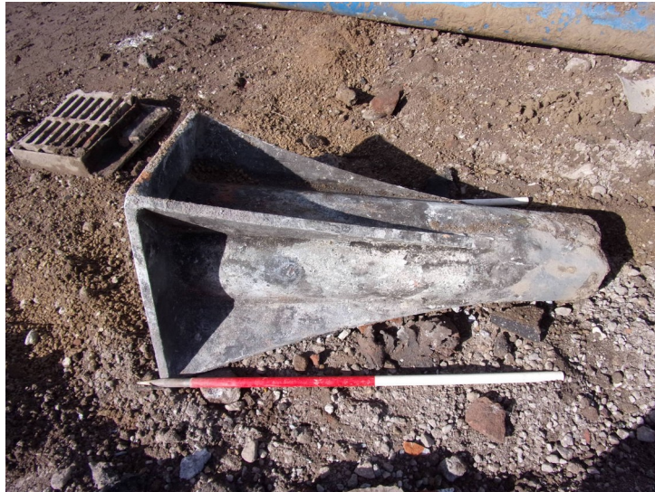
Plate 17- Cast iron fixture set within possible crane base [514], 2m scale.
