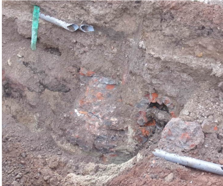
Plate 6- East facing section of brick footing [509] and associated brick tunnel [508]. Probably the remains of a dockside building which is marked as 'North Shed' on the 1893 OS map. Looking southwest.
