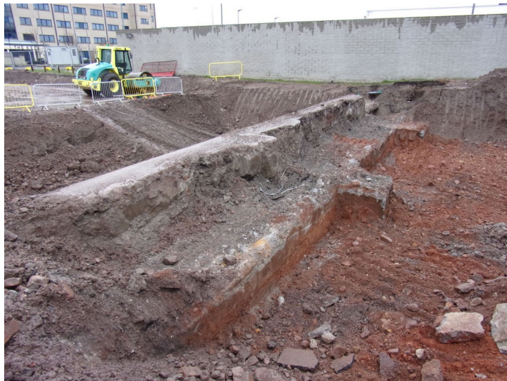
Plate 2- Concrete buttress supports [501] and red sandstone backfill deposit (502). Looking southwest.
