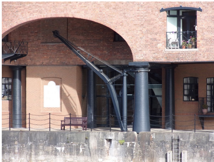
Plate 18- Example of an in situ cast iron crane set on the edge of the neighbouring Wapping Dock wall
