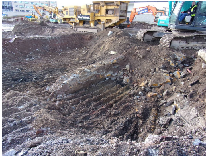
Plate 15- Concrete footing [511] in the eastern area of the site. Looking southwest.
