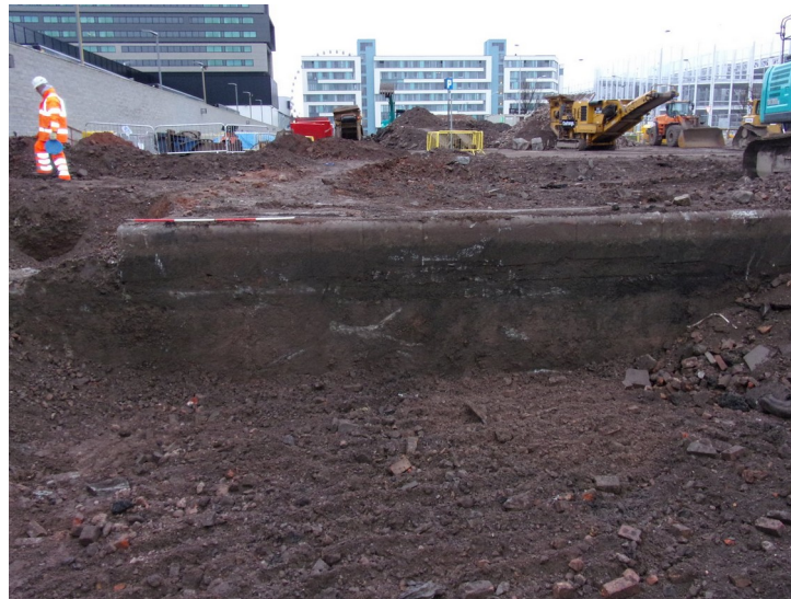
Plate 1- The southern face of the early 20 th century Queen's Branch Dock wall [500] with granite coping blocks. Looking north, 2m scale.
