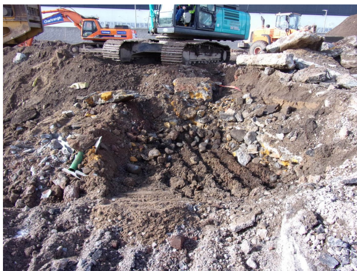
Plate 14- Mixed deposit (512) in the eastern area. Looking west.
