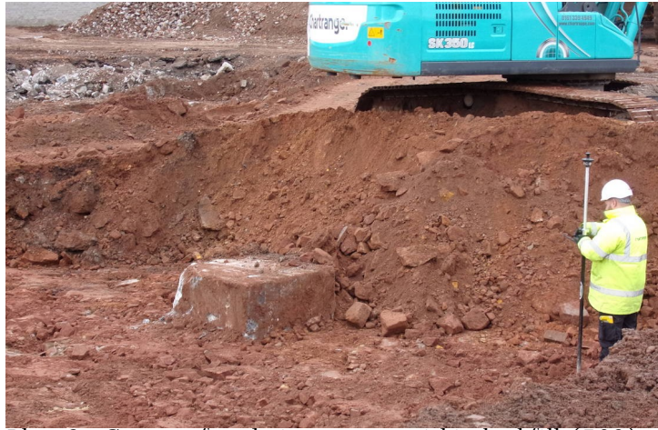
Plate 3- Concrete foundation support within backfill (502).
