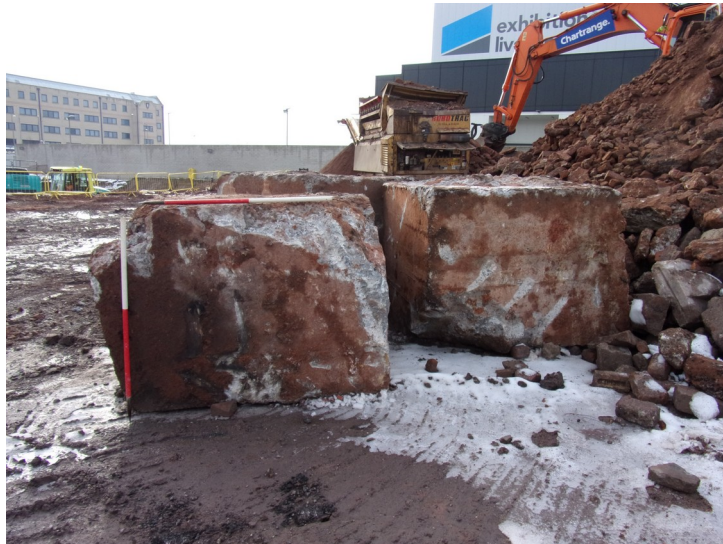
Plate 4- Concrete foundation supports after removal from (502).
