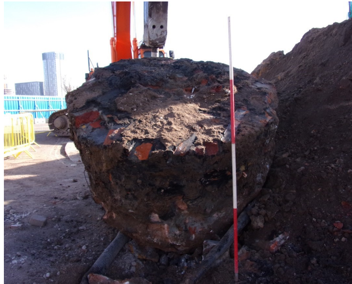
Plate 13- A possible northern Crane base after removal. Facing South.
