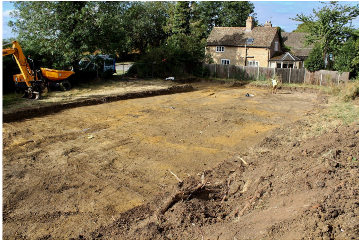
Plate 1 - Site view looking southwest.
