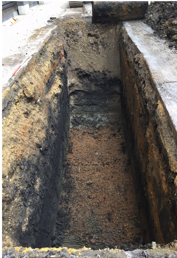
Plate 4 - TR4 under excavation. View from the north east.
