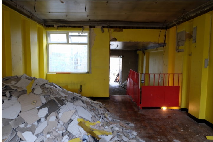
Plate 4 - Eastern room on first floor, facing west (2 x 1 m scale)
