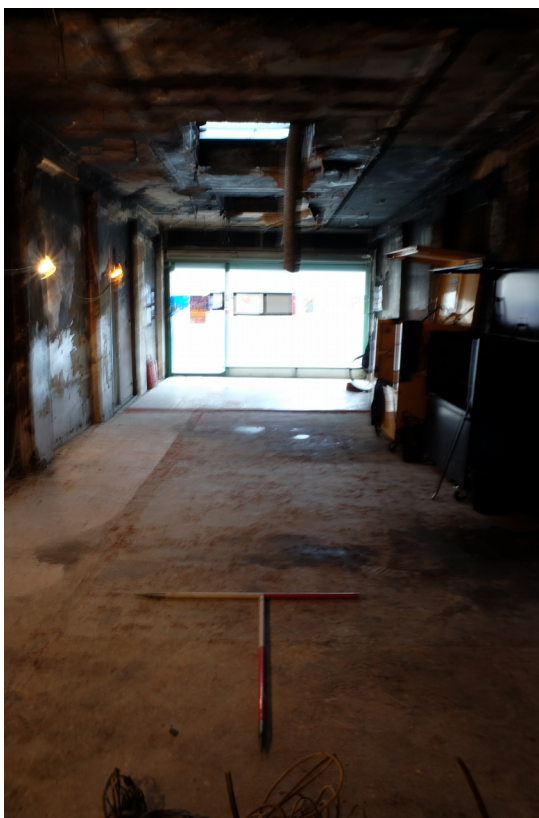
Plate 8 - Ground floor of number 57, facing east (2 x 1m scale)
