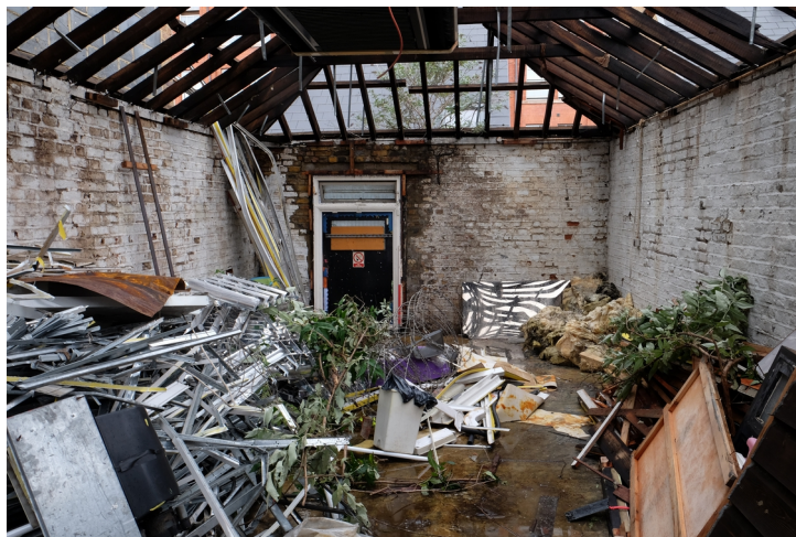
Plate 5 - West room in first floor extension (unsurveyed)
