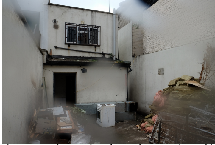
Plate 6 - Rear elevation of number 57, facing east (1m scale)
