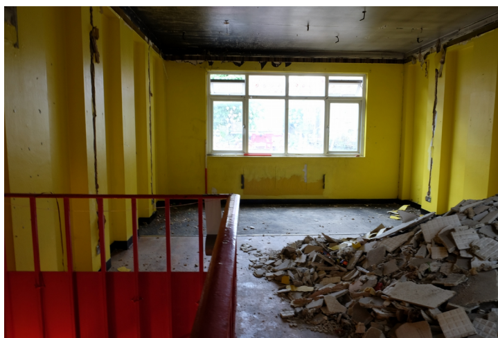
Plate 3 - Eastern room on first floor, facing east (2 x 1m scale)
