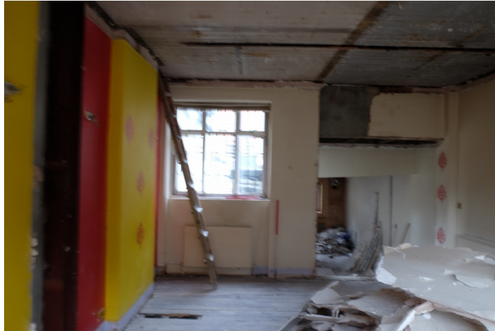
Plate 7 - First floor of number 57, facing west 2 x 1m scale)
