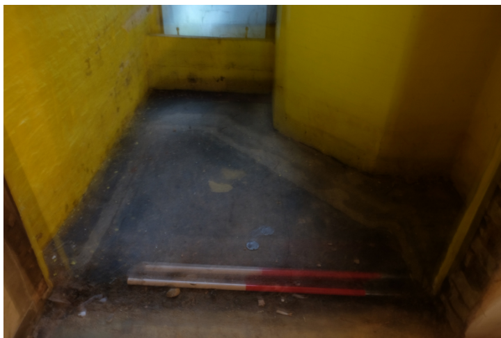
Plate 9 - Ghosting of original fireplace (1 x 1m scale)
