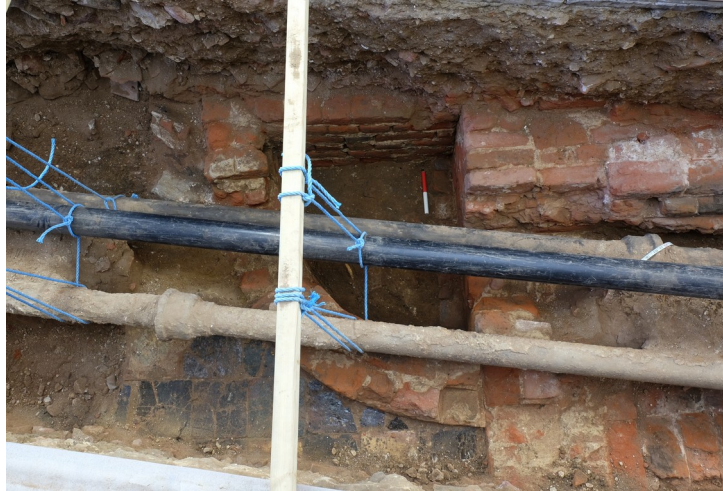
Plate 11 - Brick structure {SGR: 60} abutting the north end of the chimney breast. Photograph taken facing east, 0.2m scale.
