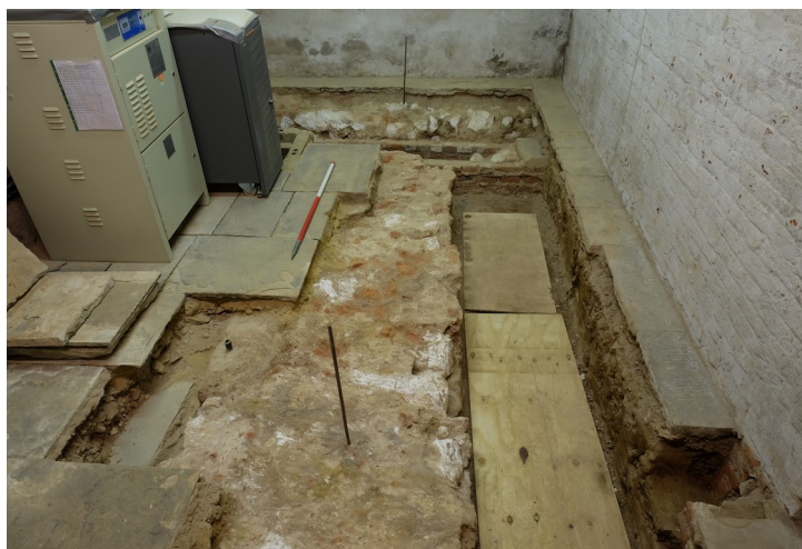
Plate 16 - Rammed chalk raft foundation below the modern floor in the Great Hall undercroft. Photograph taken facing east, 1m scale.
