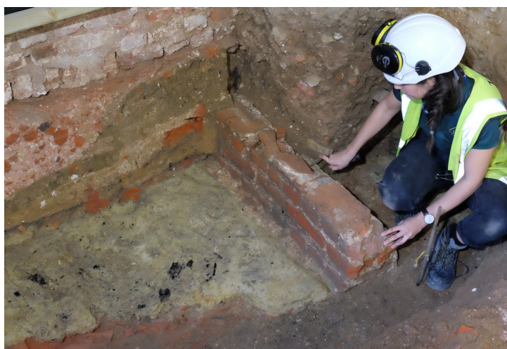
Plate 14 - Truncated remains of north-south wall {SGR: 30}. Photograph taken facing north-east, working shot featuring Florence Laino.
