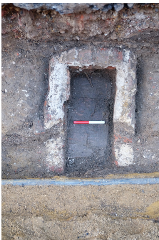
Plate 4 - Culvert {SGR: 16} with the roof removed. Photograph facing north, 0.2m scale.
