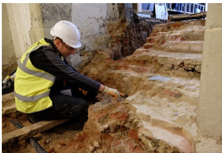
Plate 19 - The stairs {SGR: 70} were built from a foundation of bricks with reigate stone treads. Photograph taken facing north-west, working shot featuring Daniel Bateman.
