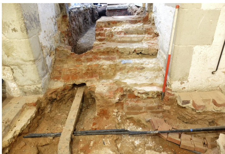
Plate 18 - Remains of the brick staircase {SGR: 70}. Photograph taken facing north, 1m scale.
