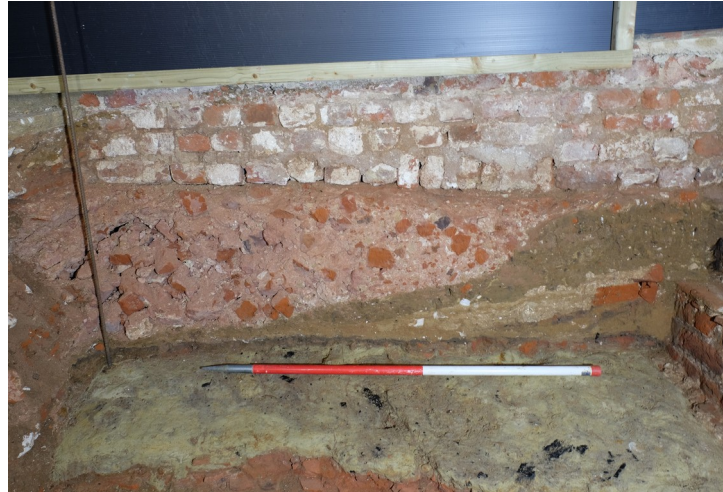
Plate 15 - The build up of layers {SGR: 33} to construct the Henrician extension of the kitchens. Photograph taken facing north, 1m scale.
