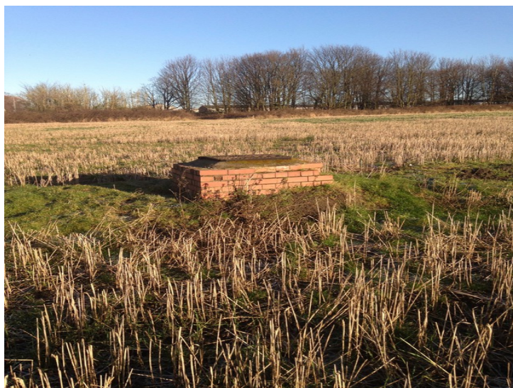
Plate 17 - Brick manhole to the western side of site 2. Looking north-northeast.
