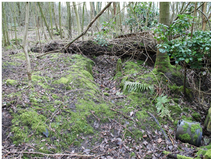
Plate 7 - Possible culvert feature in southeast area of site 1, facing south.
