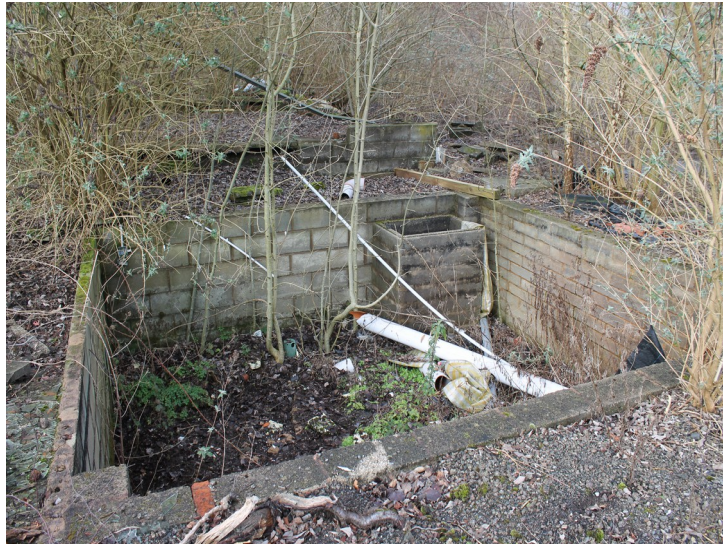
Plate 5 - Sunken breeze block chambers.
