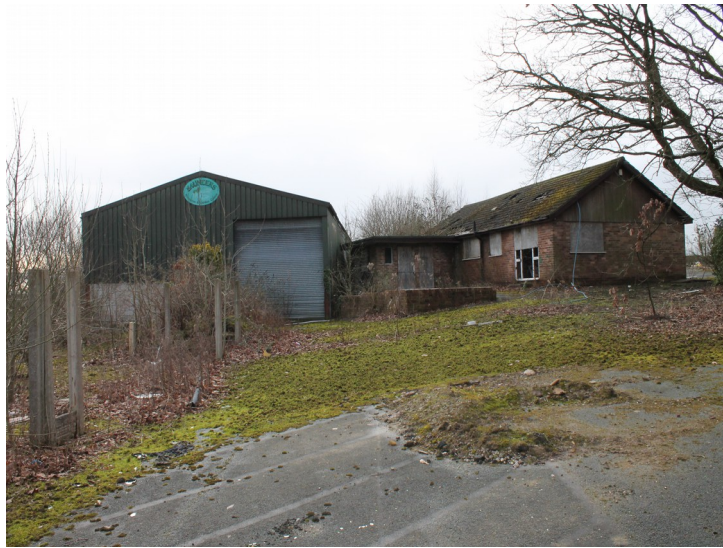
Plate 1 - Extant buildings at site 1, facing south.
