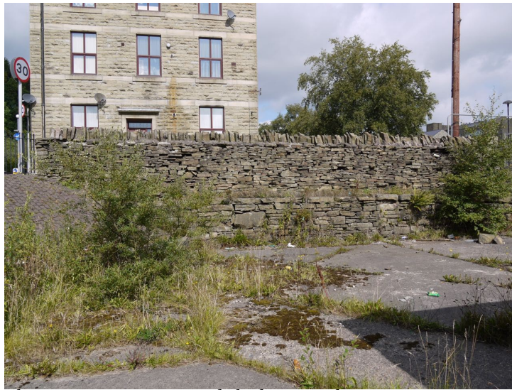
Plate 27: Lower courtyard, looking north to Henrietta Street
