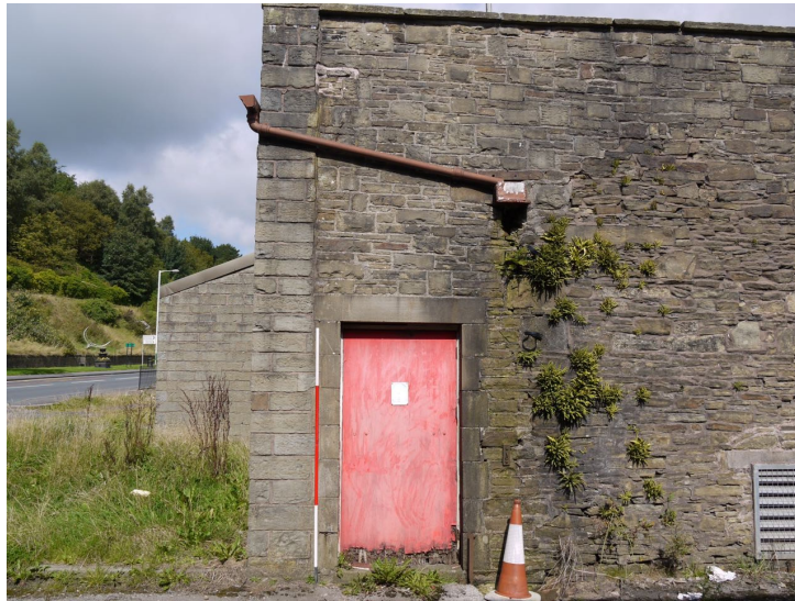
Plate 25: Southern elevation of extension A2
