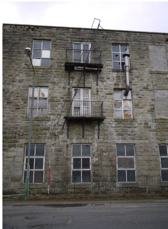
Plate 6: Fire escape on the northern elevation
