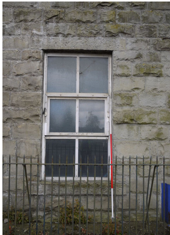
Plate 3: Window form, northern elevation
