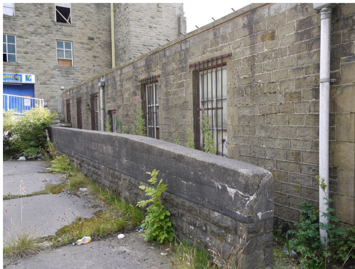
Plate 29: North elevation of extension C
