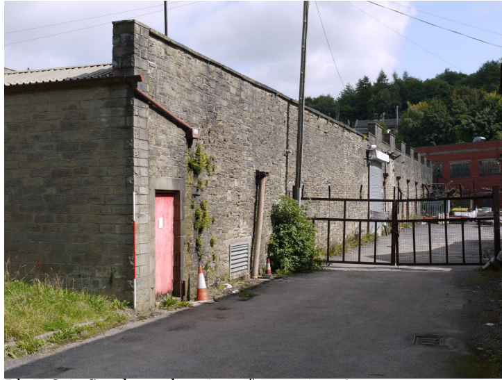
Plate 24: Southern elevation of extension A
