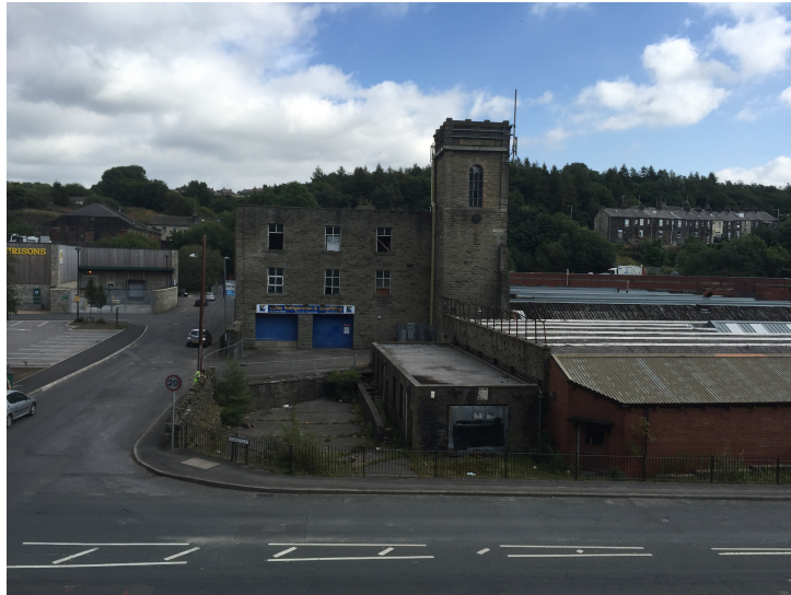
Plate 15: Western elevation of water sprinkler tower
