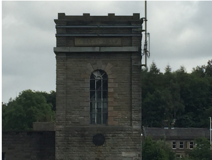
Plate 18: Third floor of the water sprinkler tower
