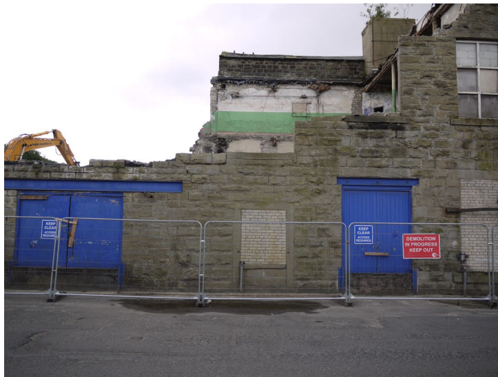
Plate 9: Eastern section of the northern elevation, showing modifications
