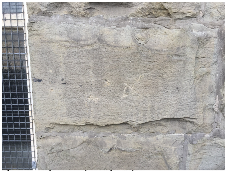
Plate 7: Markings on the northern elevation
