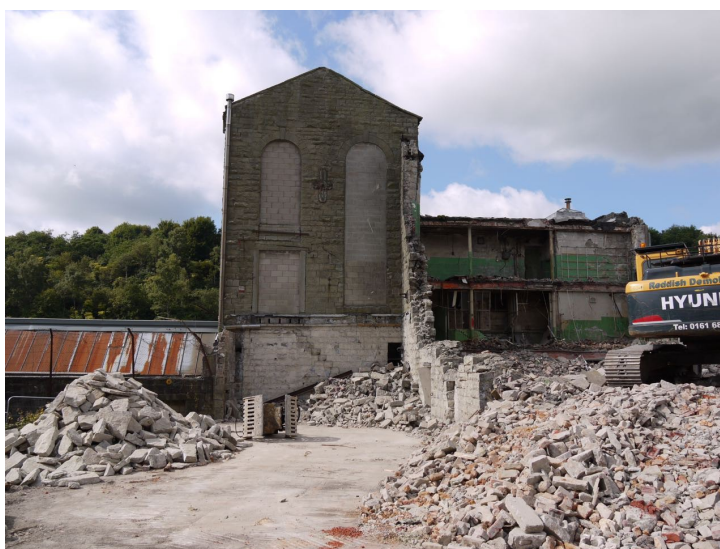
Plate 20: Eastern elevation of the engine house
