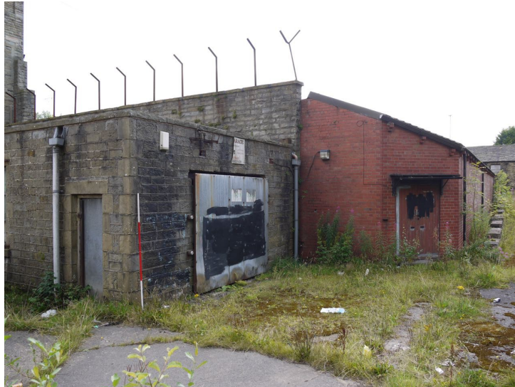
Plate 28: Junction of extension C and E, looking south
