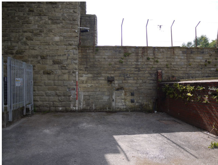
Plate 16: Wall for the southern extension, as viewed from the courtyard
