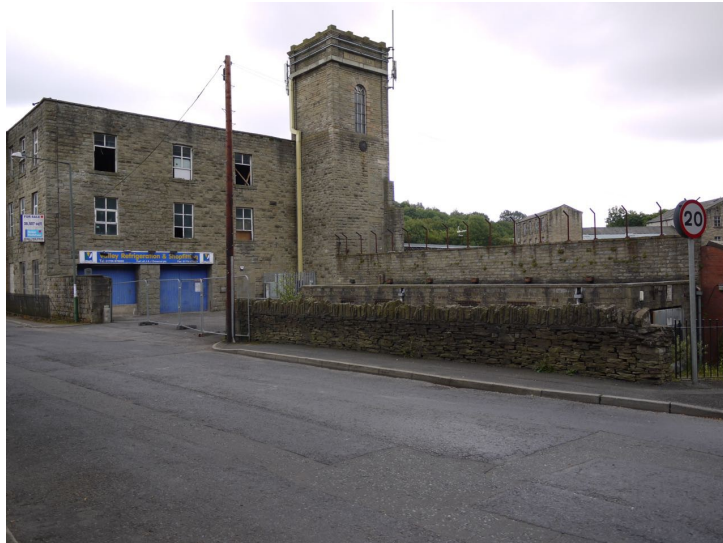
Plate 12: Western elevation of the mill
