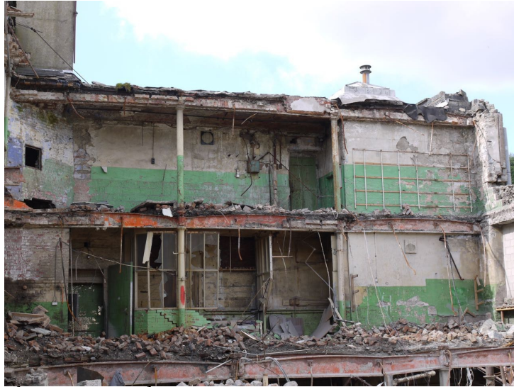
Plate 21: Exposed eastern cross section
