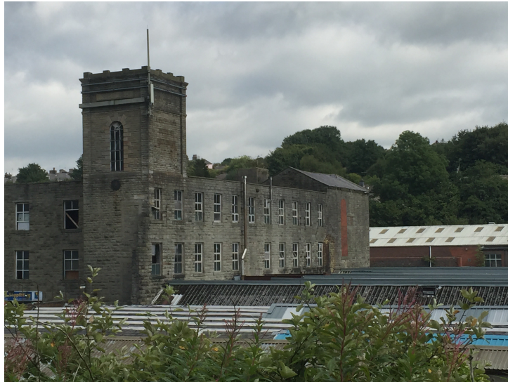
Plate 19: Southern elevation of the mill
