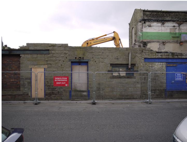
Plate 10: Blocked arches on the northern elevation
