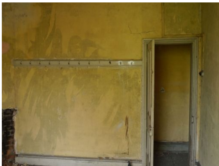
Plate 18: Southern room of second floor
