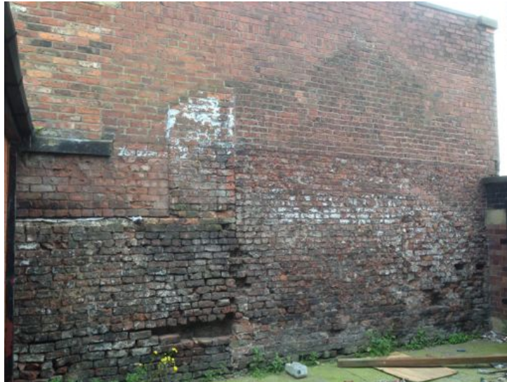
Plate 11: Boundary wall of Dog and Duck and Abbey Inn, looking southwest
