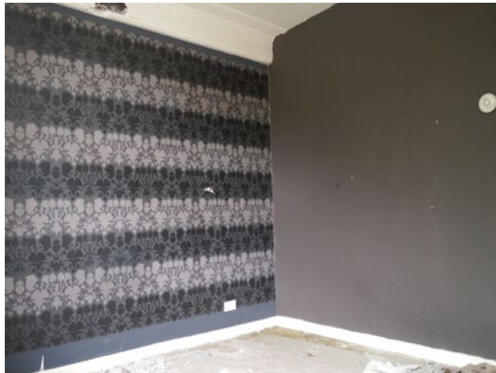
Plate 16: Northeast room of first floor, showing cornice
