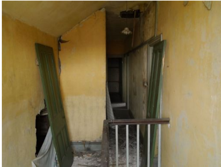
Plate 17: Second floor corridor
