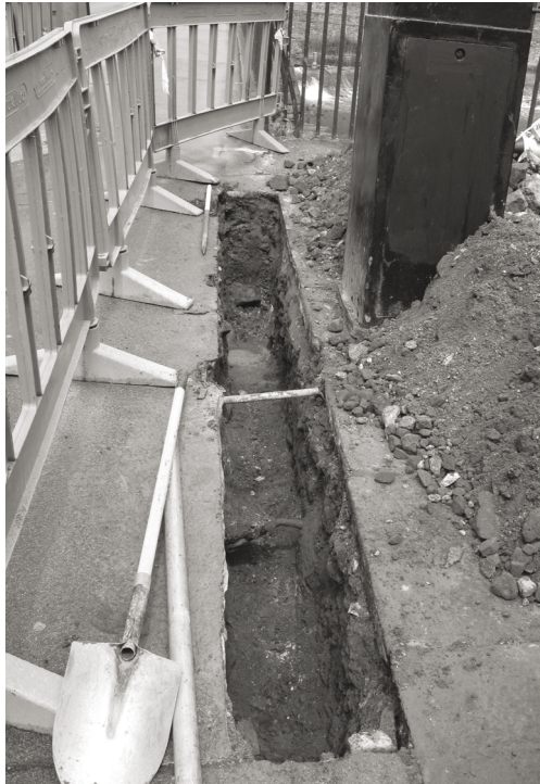
Plate 2 - Trench looking northwest. showing services within the trench. Scale 1m
