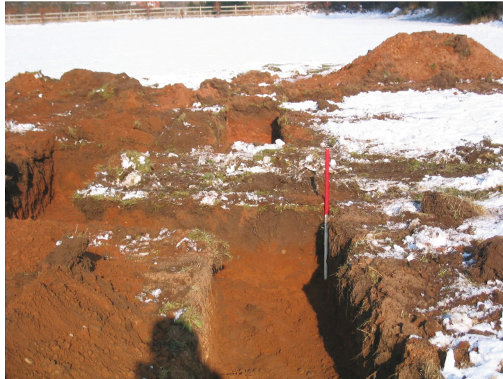
Plate 2 - South facing section of footing excavations, 1m scale
