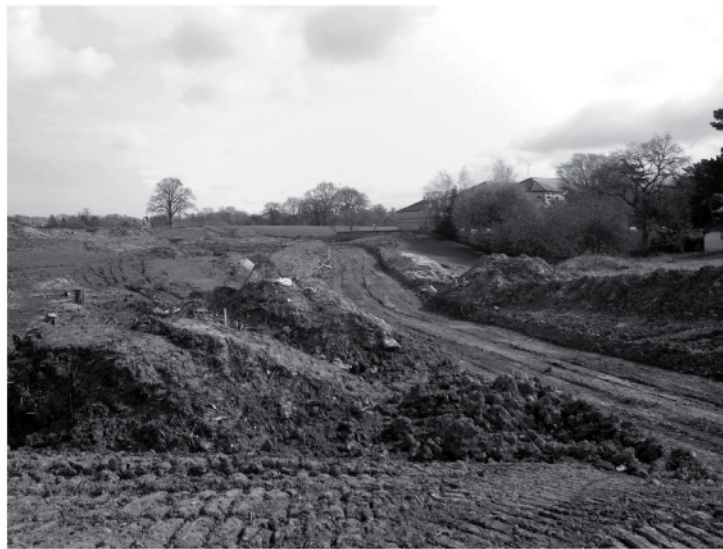
Plate 1 - North of Brook Lane. Facing North
