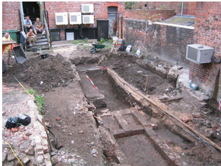
Plate 1 - Excavation area, looking east
