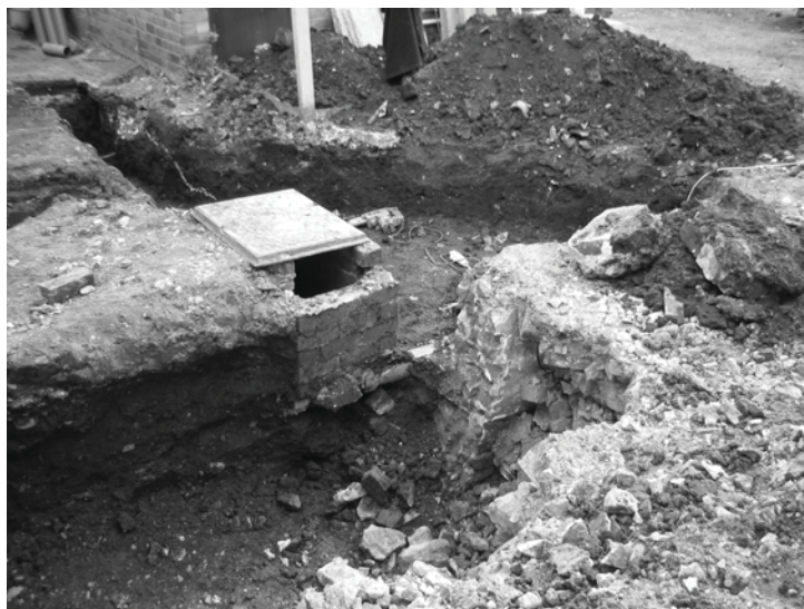
Plate 6 - Excavation for bin store showing rubble (34), looking southeast
