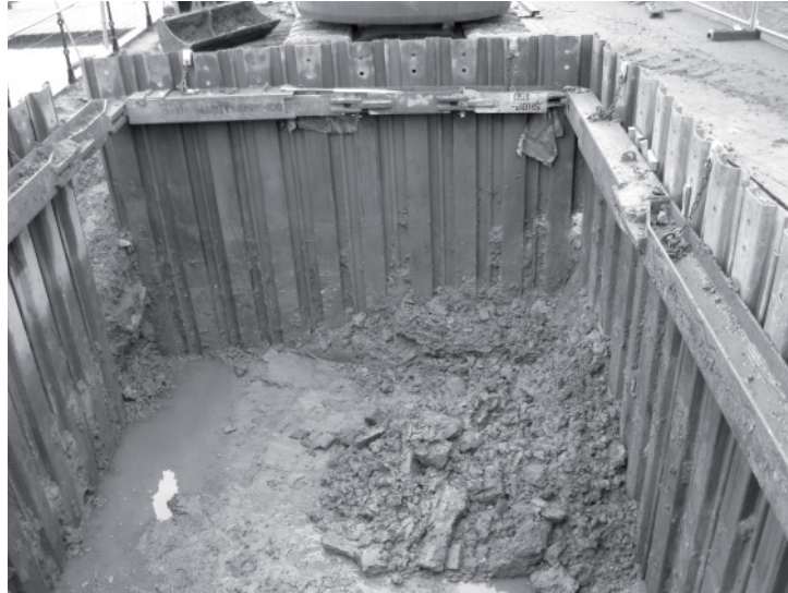
Plate 1 - View of excavated area at maximum depth, looking west
