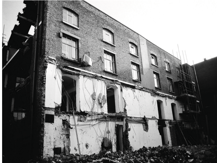
Plate 2 - West elevation revealed after demolition of 20th century additions.
