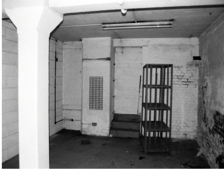
Plate 11 - View of the south wall of B.9, note the brick pier, blocked doorway and concrete column detail.
