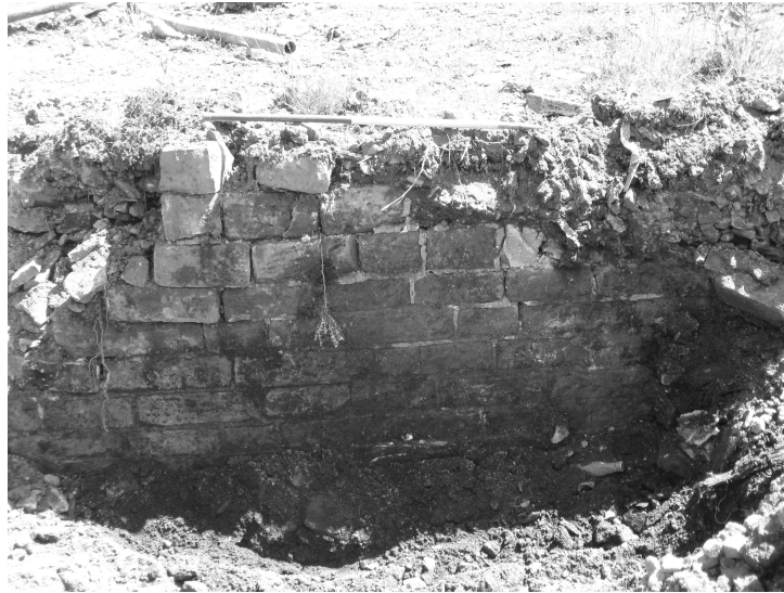
Plate 10 - Wall 906 facing southeast. Scale 1m.
