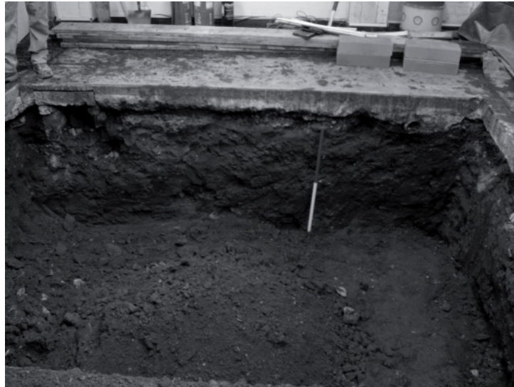
Plate 4 - Lift Shaft excavation facing east, scale 1m
