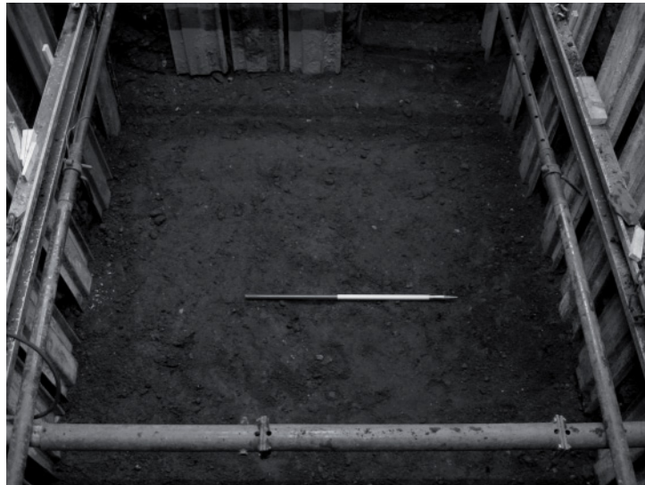
Plate 5 - Lift shaft excavation facing south, scale 1m
