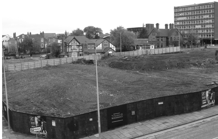
Plate 1 - Site area following topsoil strip, looking north
