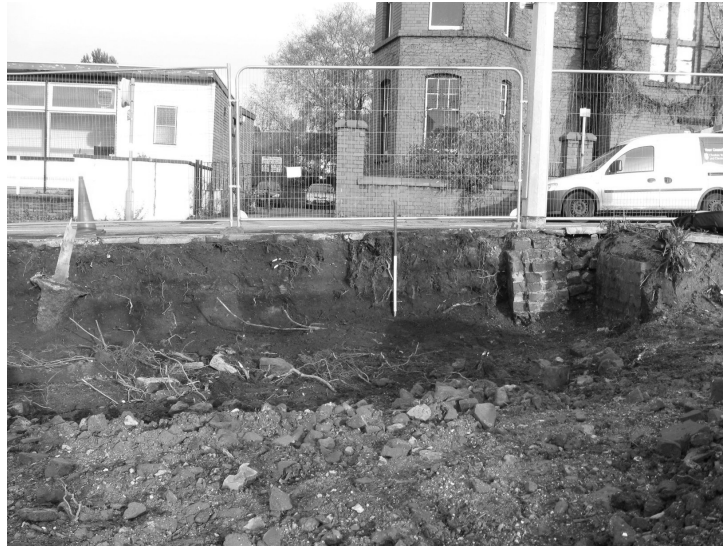
Plate 3 - Hunter Street section, looking north. 1m scale
