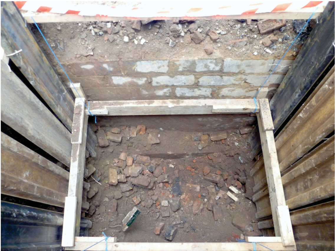
Fig 5 Trench west of cellar looking east
