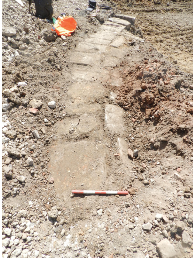
Fig 6 Nineteenth to twentieth century surface in Phase 2 area, looking west, 0.5m scale
