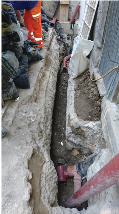
Fig 5 Excavated drain run looking north
