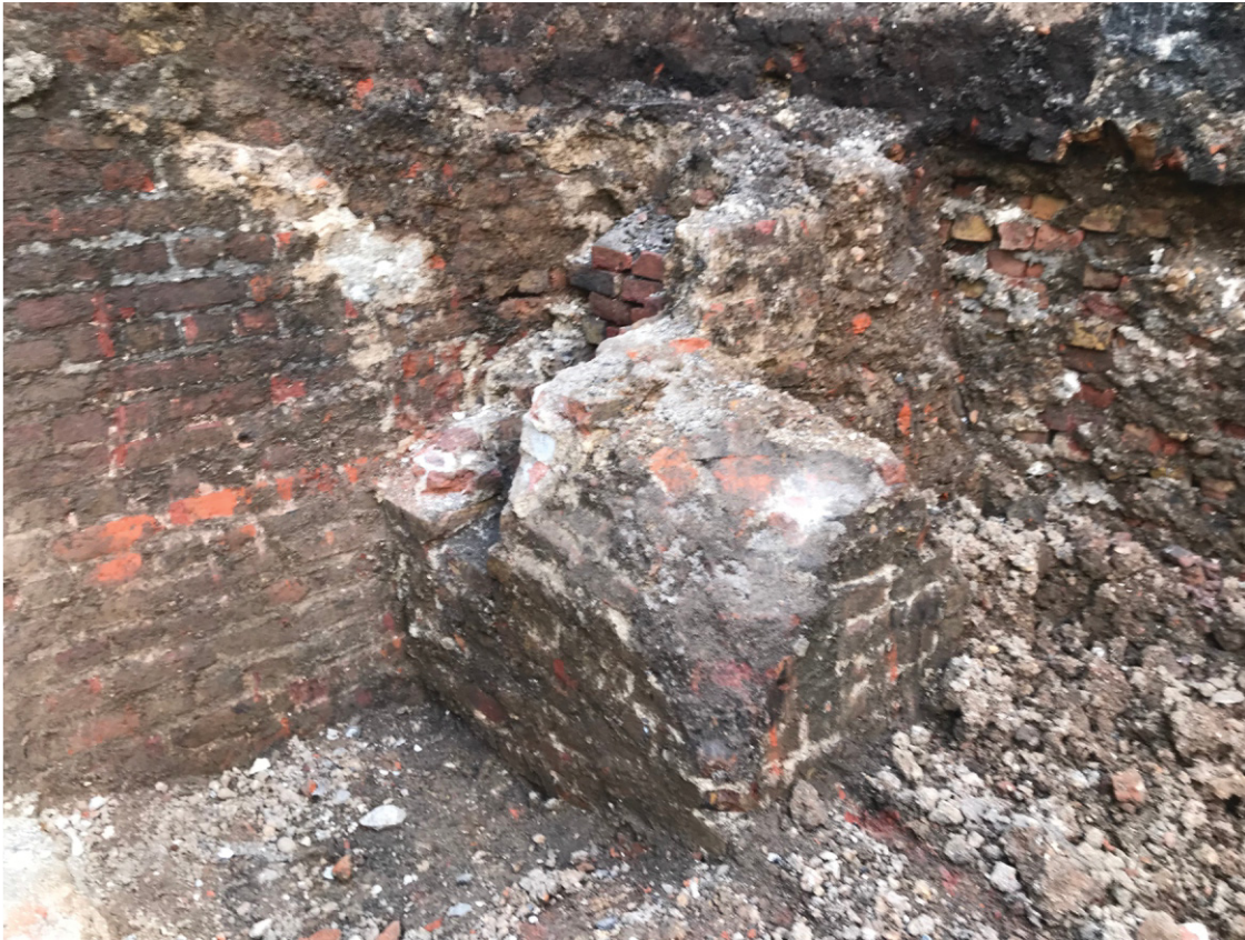
Fig 4 Brick wall in north-eastern area
