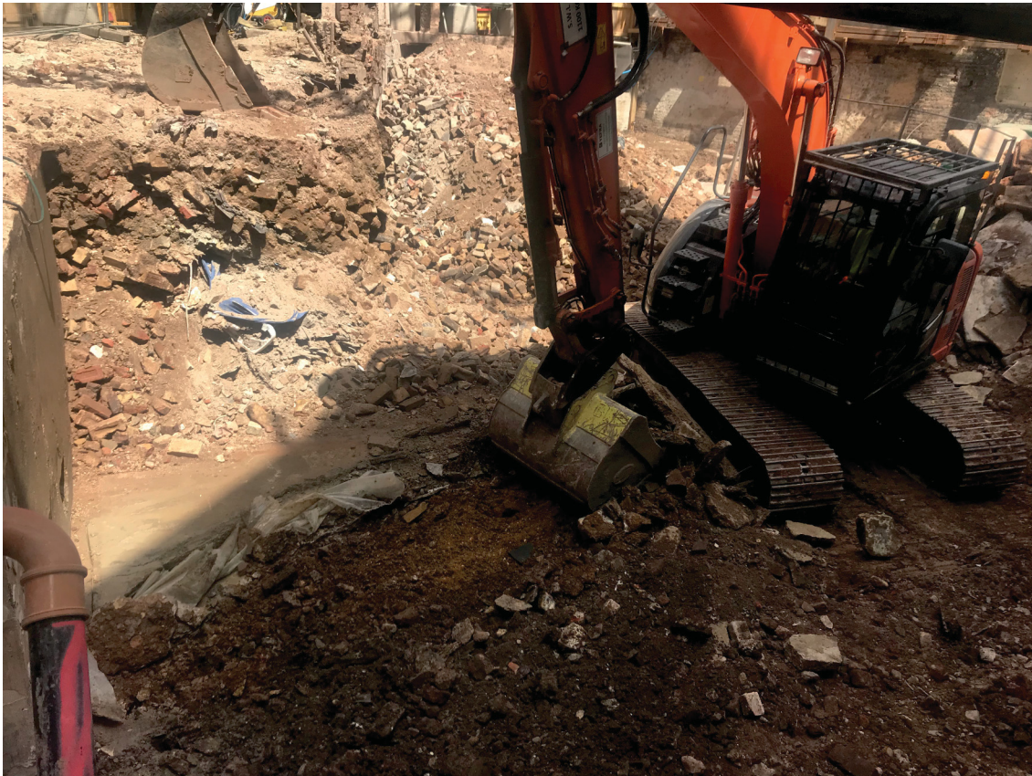
Fig 6 Concrete slab and its formation layers in southern area
