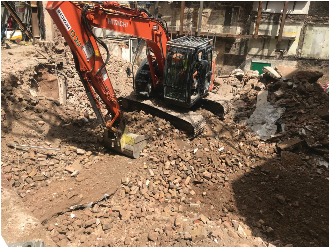
Fig 5 General demolition (brick) rubble
