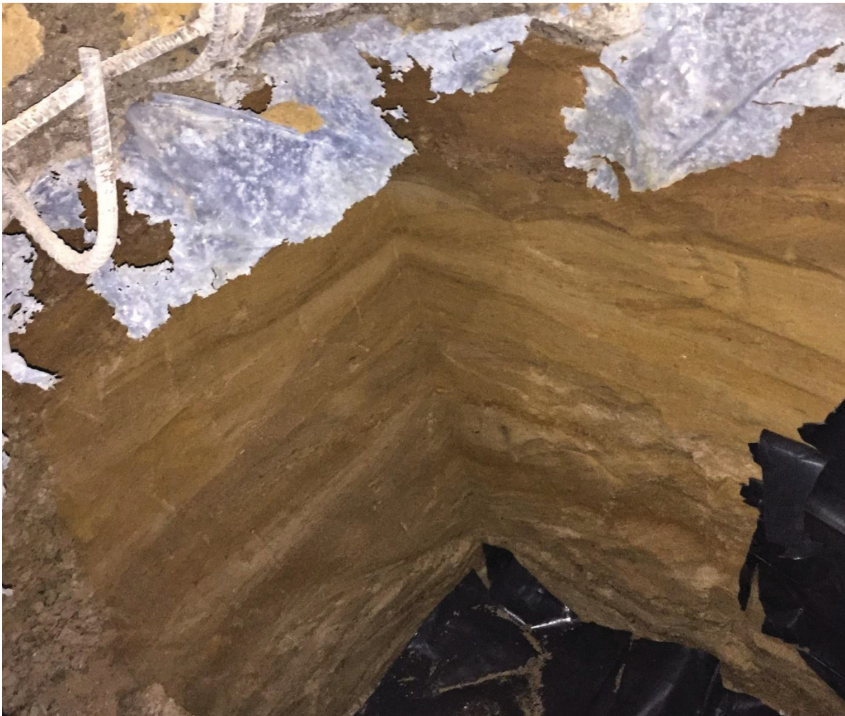
Photo 1 U-pin hole, looking west
