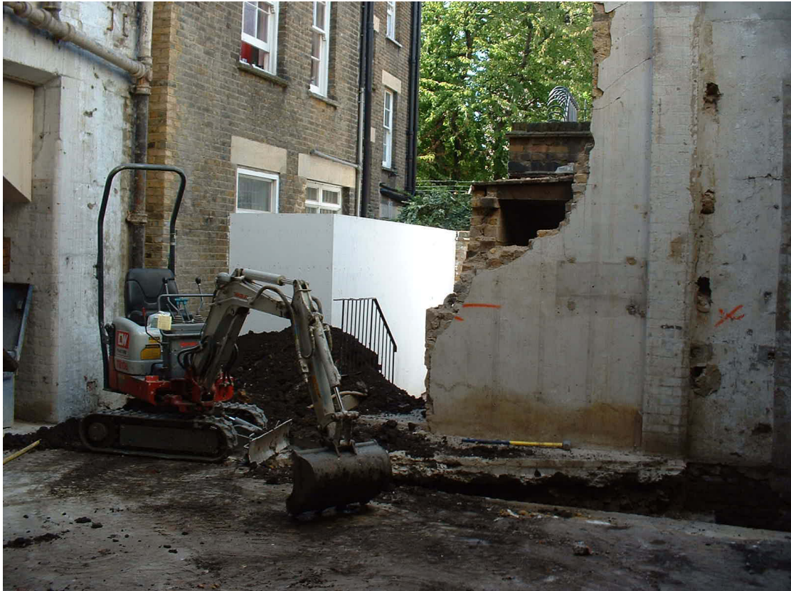
General view: digging the drains
